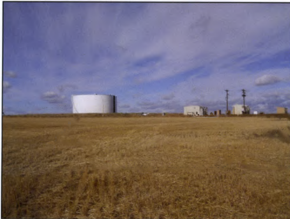
Figure 5. Northern reroute area showing existing infrastructure in the background, view to the northwest.
