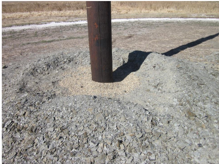
Photo 14. Example post hole filled with aggregate. Shale surrounding the hole was debris from underlying material as a result of post hole drilling. Upon final restoration, material will be cleaned, spread, or hauled away.
