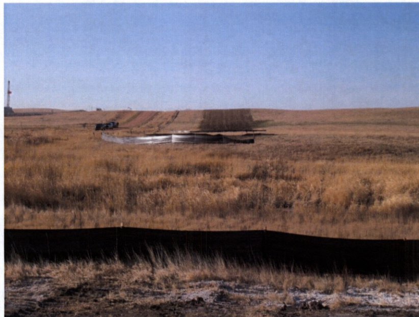
Photo 10. Direction: South. Photo shows pipeline right-of-way where it bores underneath a wetland at observation point 128 ( Figure 1 ). Erosion control structures were in place and no erosion to the water body was evident.
