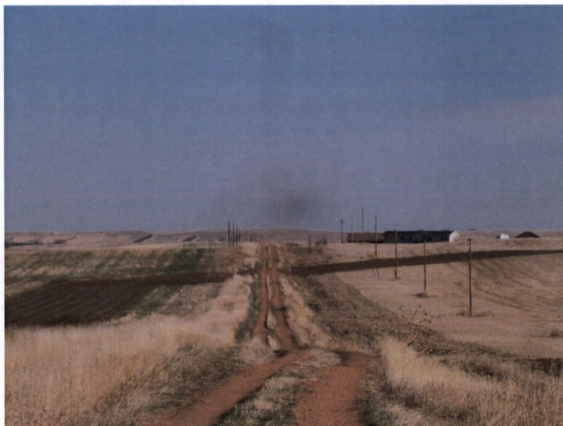
Photo 18. Direction: North. Photo shows where pipeline right-of-way bores under 124 th Avenue. From this point, the right-of-way parallels the existing Bridger Pipeline to the Skunk Hill Station.
