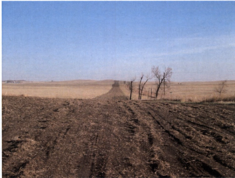
Photo 3. Direction: North. Same location as Photo 2. This photo shows the right-of-way for the Whiting Pipeline. At the time of our site visit the right-of-way needed final seeding and restoration
