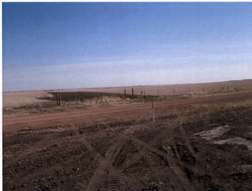
Photo 20. Direction: Northeast. This photo shows the right-of-way of the Whiting Pipeline where it bores under 28 th Street. Fence in background was repaired and in working condition. Cathodic tester is barely visible to the right of gate (orange pole).
