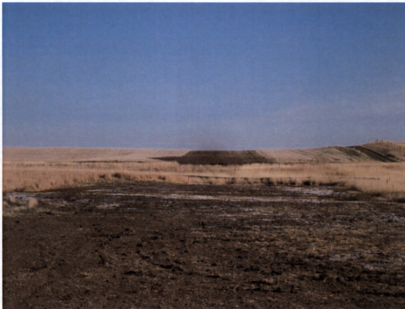
Photo 14. Direction: North. Photo shows pipeline right-of-way where it bores underneath a wetland less than 0.25 miles north of observation point 131. Erosion control structures were in place and no erosion to the water body was evident.
