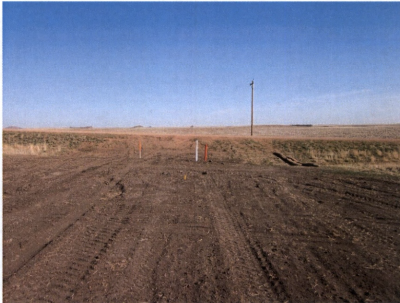
Photo 17. Direction: North. This photo shows the right-of-way of the Whiting Pipeline where it bores under 30 nd Street. No erosion or other issues were noted. Example cathodic tester indicated by the orange pole; testers were located at every mile along pipeline ROW.
