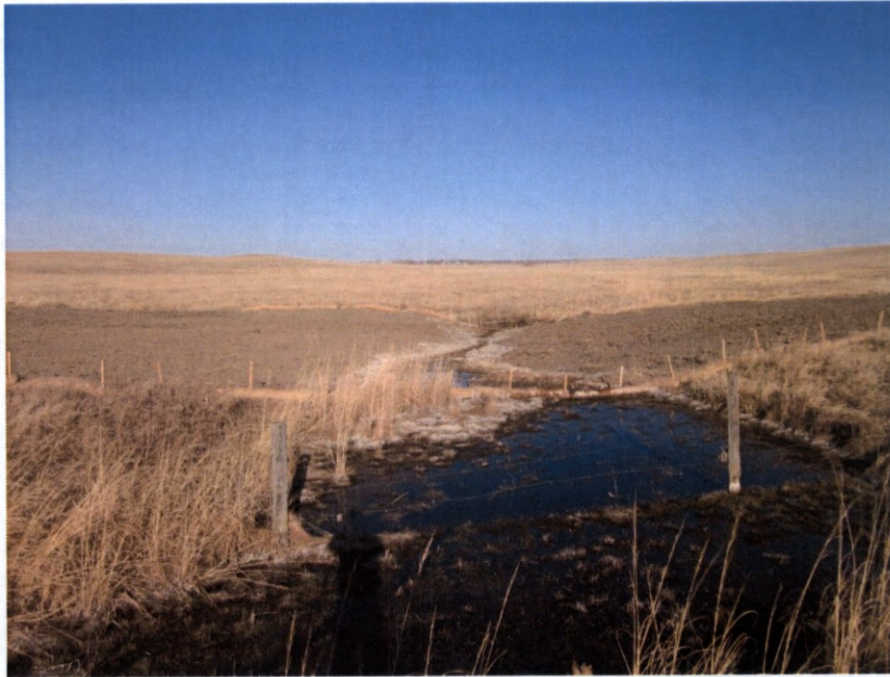
Photo 7. Direction: West. Erosion control structure located along pipeline right-of-way. No erosion or sedimentation was noted within the water body.
