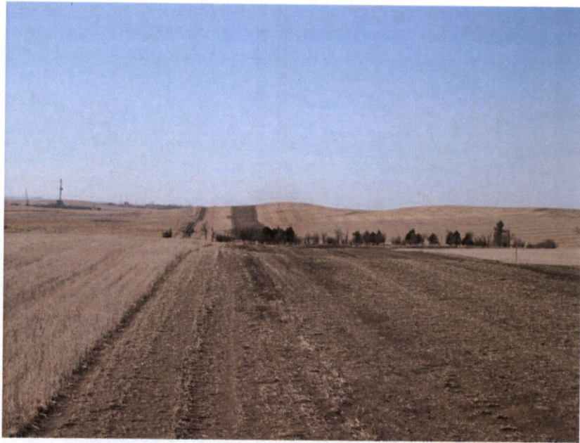
Photo 15. Direction: South. Photo shows pipeline right-of-way north of where the pipeline bores under the tree row and about a quarter mile south of 30 th Street.
