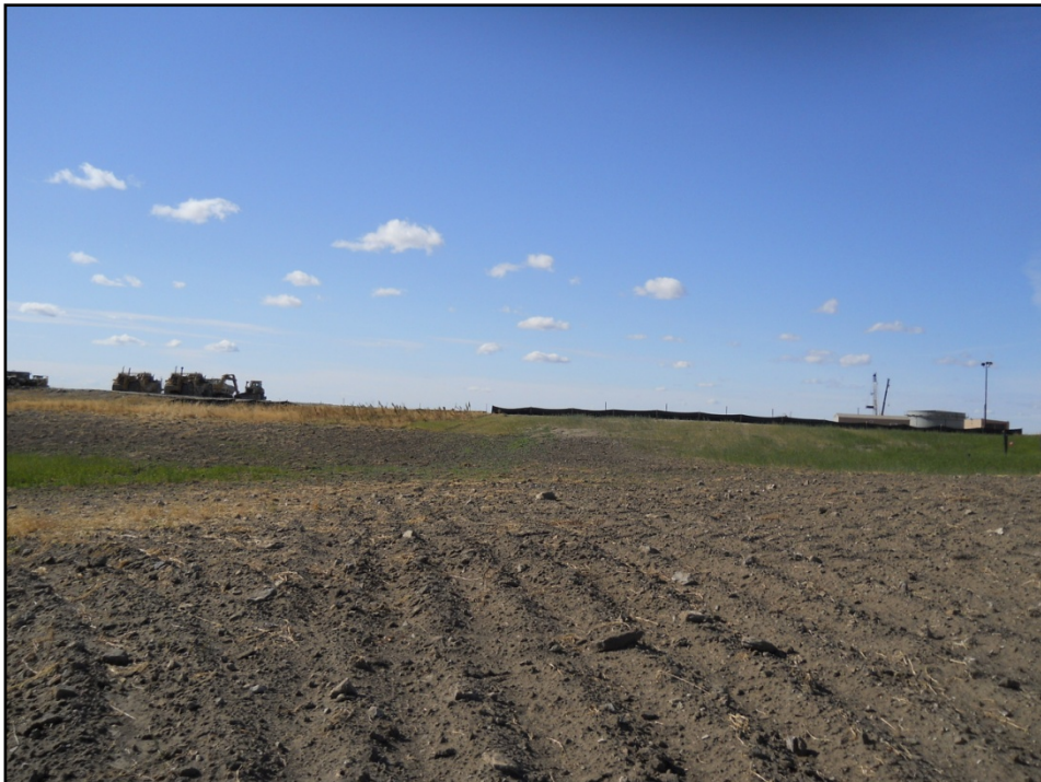
Figure 8. Southern reroute overview, showing existing infrastructure in the background, view to the west.
