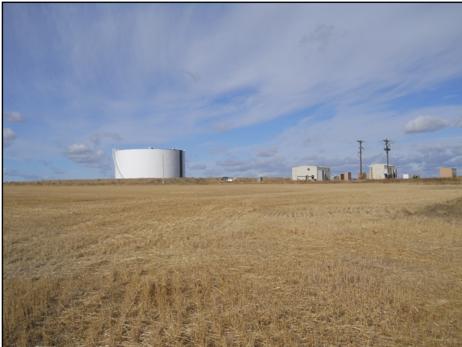
Figure 5. Northern reroute area showing existing infrastructure in the background, view to the northwest.
