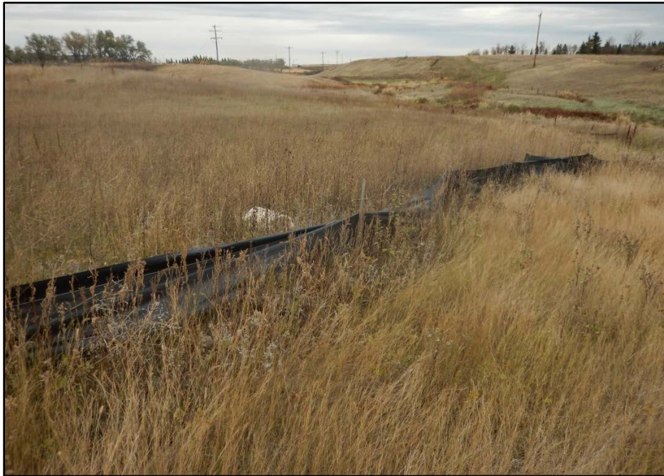
Figure 5. Riparian/wetland area crossing. Directionally drilling was used to avoid impacts to this area. Wooden matting was laid upon the surface for equipment movement along the ROW during construction and had been removed. Riparian vegetation has rebounded to pre-disturbance condition and the seeding of the ROW above the crossing has reestablished to greater than 70% coverage.
