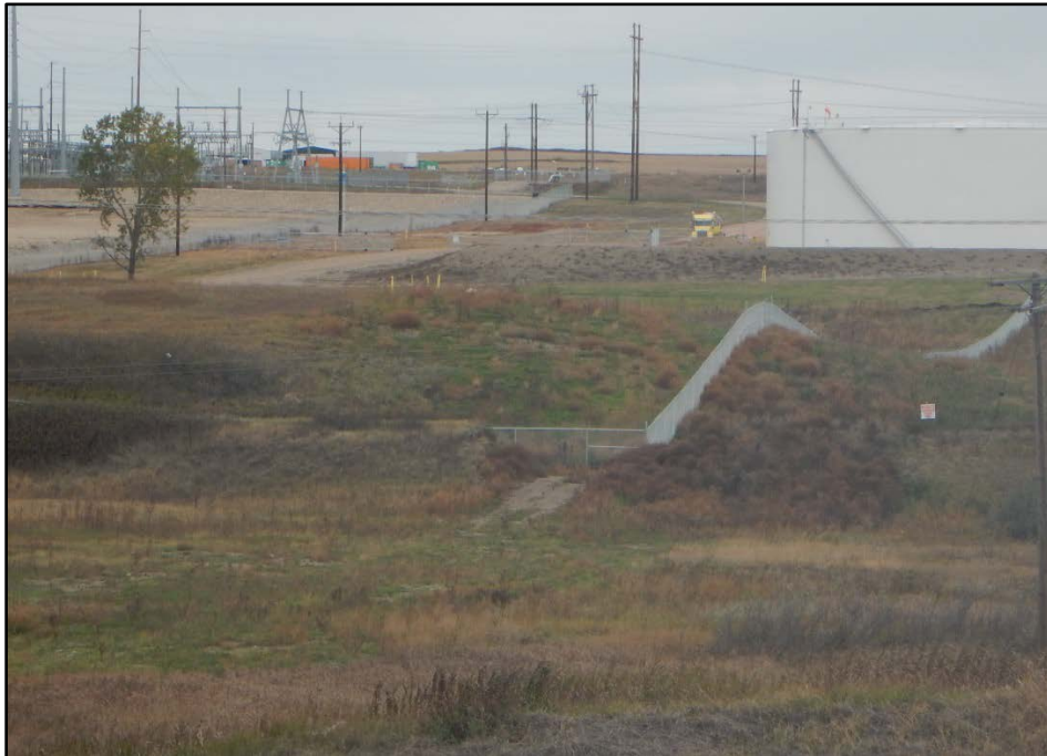
Figure 1. Pipeline ROW exiting the Hess Tioga Gas Plant. Seeded grass is becoming established and Hess will continue to monitor seeded areas.
