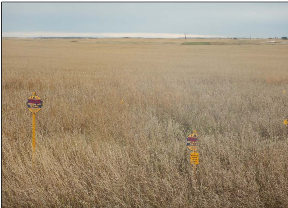
Figure 2. Reclaimed ROW within cultivated agricultural field. In 2014 the area was planted with spring wheat. Crop productivity did not seem to be negatively affected and no trench subsidence was evident.
