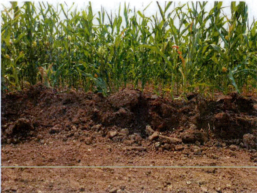
August 17 - Topsoil stripping at MP10.83 in corn field.
