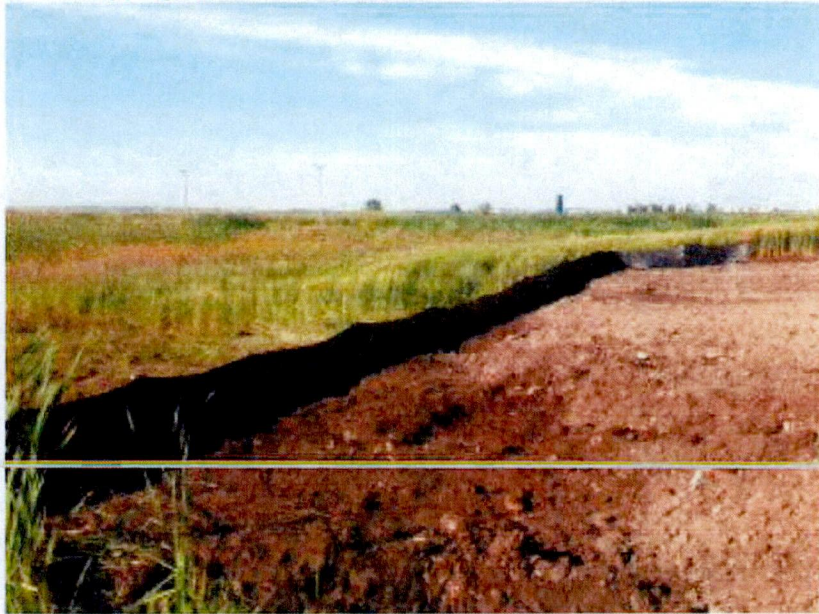
Photo 3 - Silt fence installation along adjacent wetland area.
