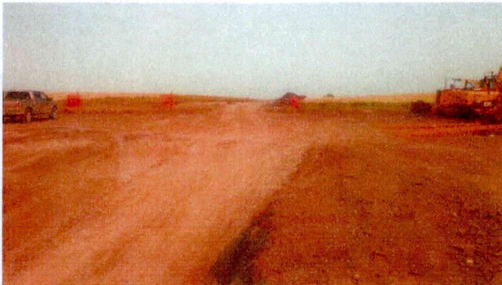
Photo 1 – Grading and stripping at startup 14+72 looking north.
