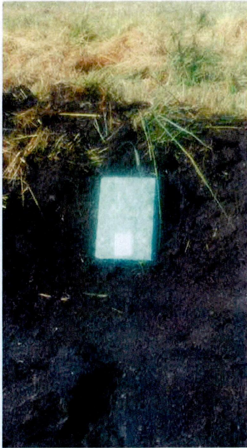
Photo 2 – Top soil stripping approximately 12 inches.
