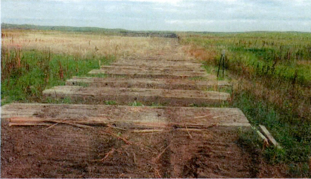
August 20 - matting places at wetland crossing in bore location at MP25.59.
