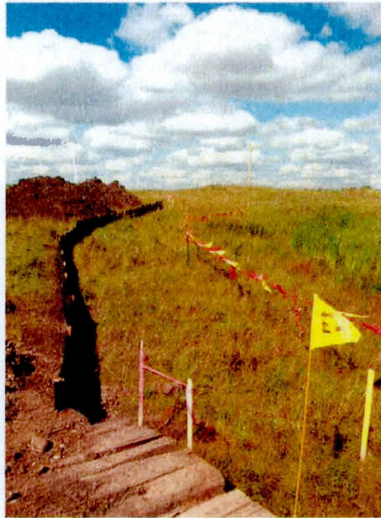
Photo 4 – Silt fence tie in to timber matting.
