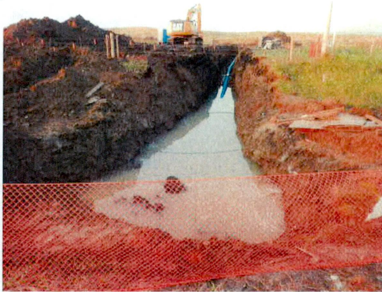
August 25 – Water collected in a boring pit and trench.
