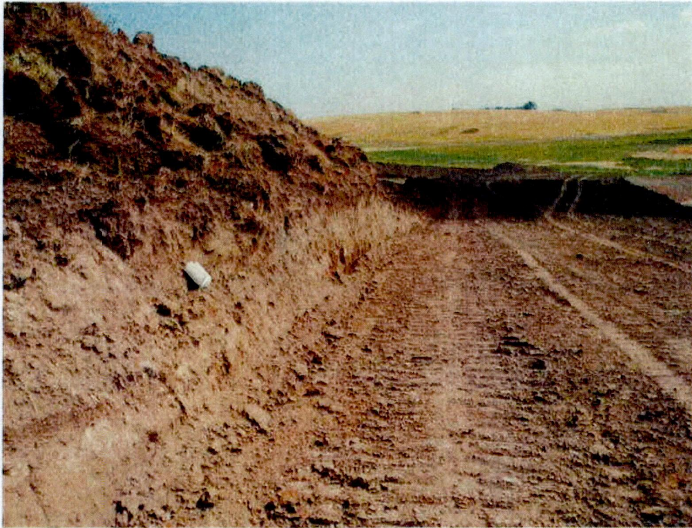
August 28 - Topsoil segregation, grading, and subsoil leveling.
