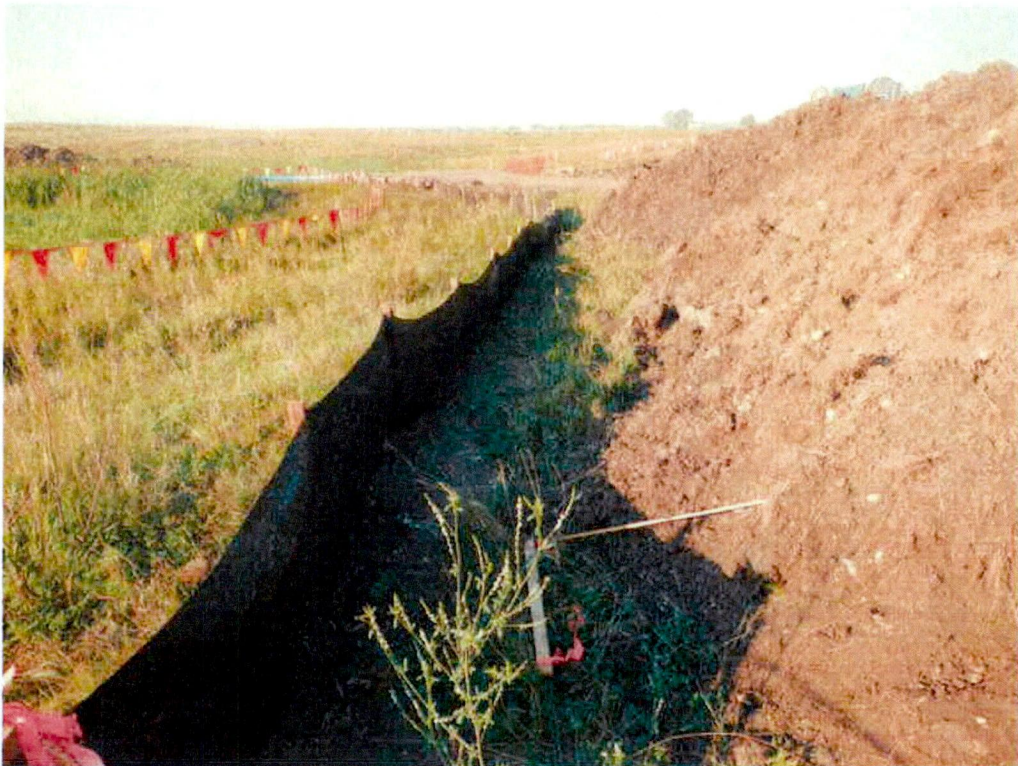
August 25 – Topsoil stockpile near a wetland protected by silt fence.
