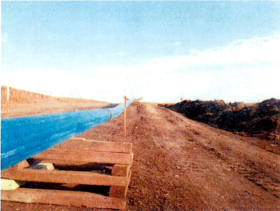
September 5, 2013 – Pipe stringing and welding at MP 0.54
