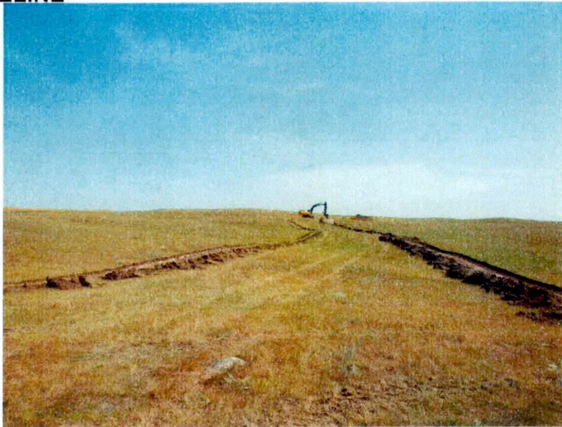
September 3, 2013 – Stripping activities near MP43.03
