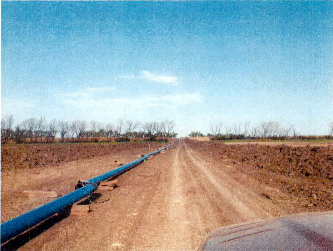
September 4, 2013 – Several shelter belts shown with pipe stringing.
