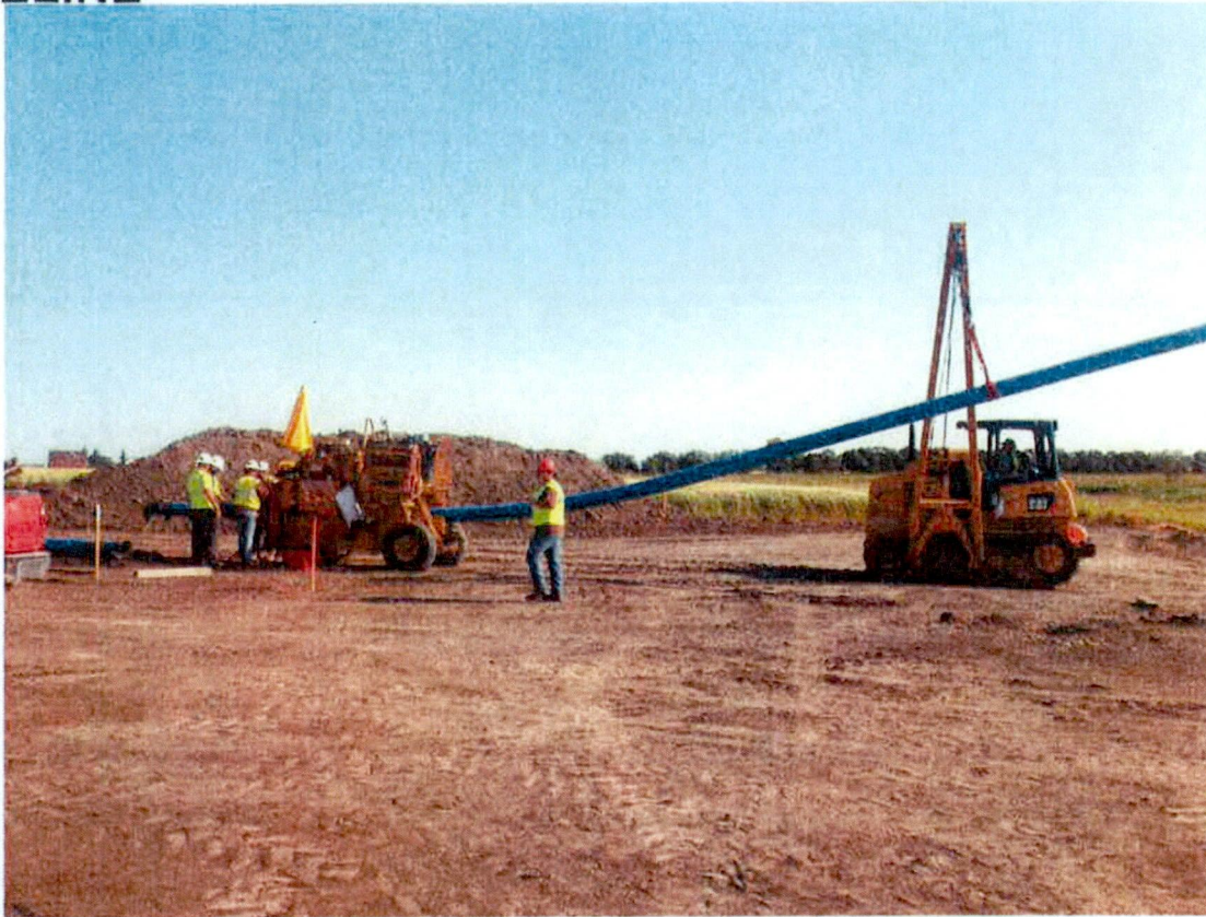
September 5, 2013 – Pipe bending operation at MP 12.03
