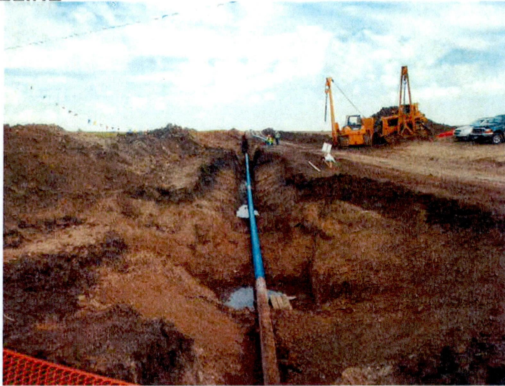
September 14, 2013. Pipe Stringing
