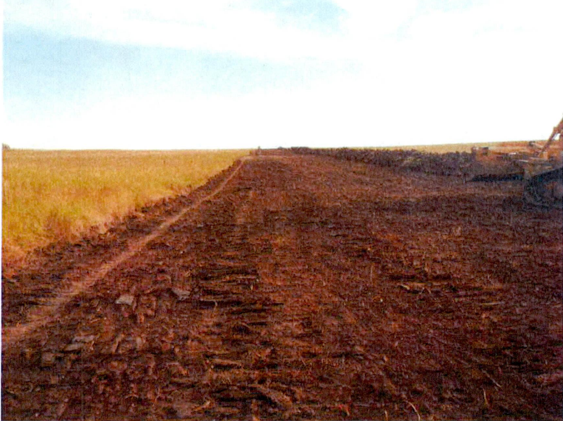
September 14, 2013 – Stripping activities near MP61.25
