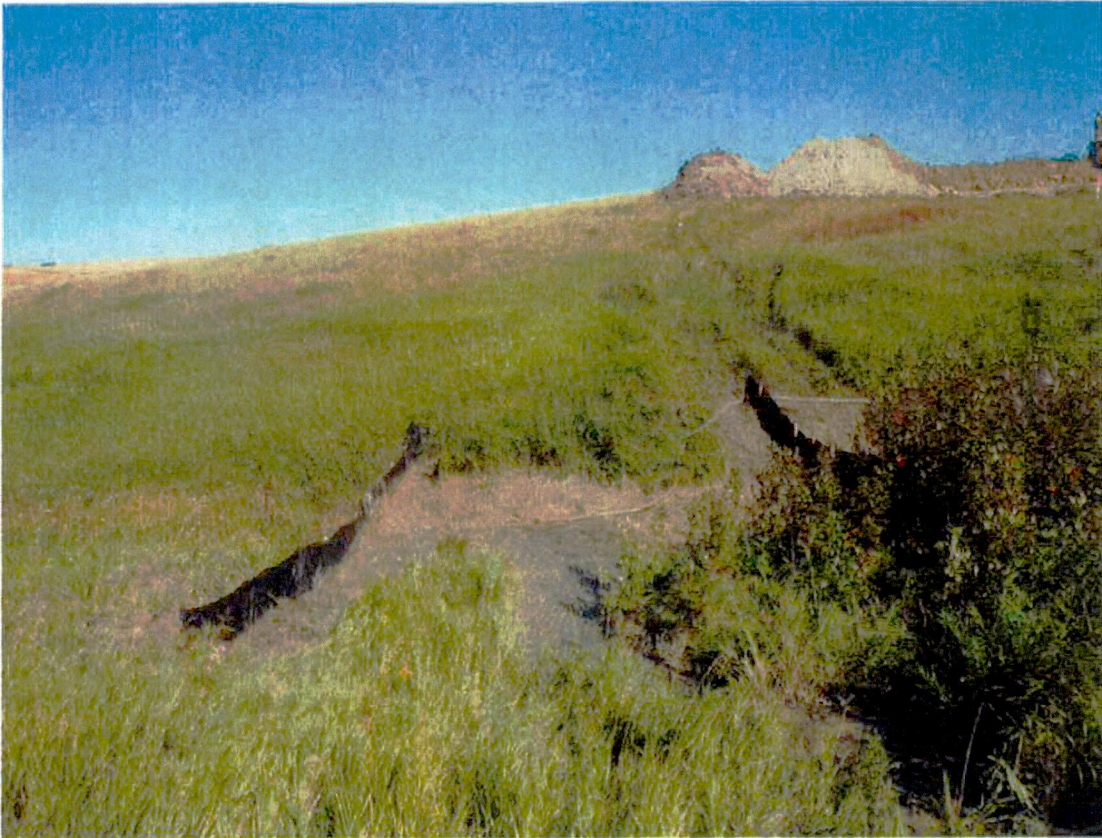
September 12, 2013 Silt fence containment of frac-out
