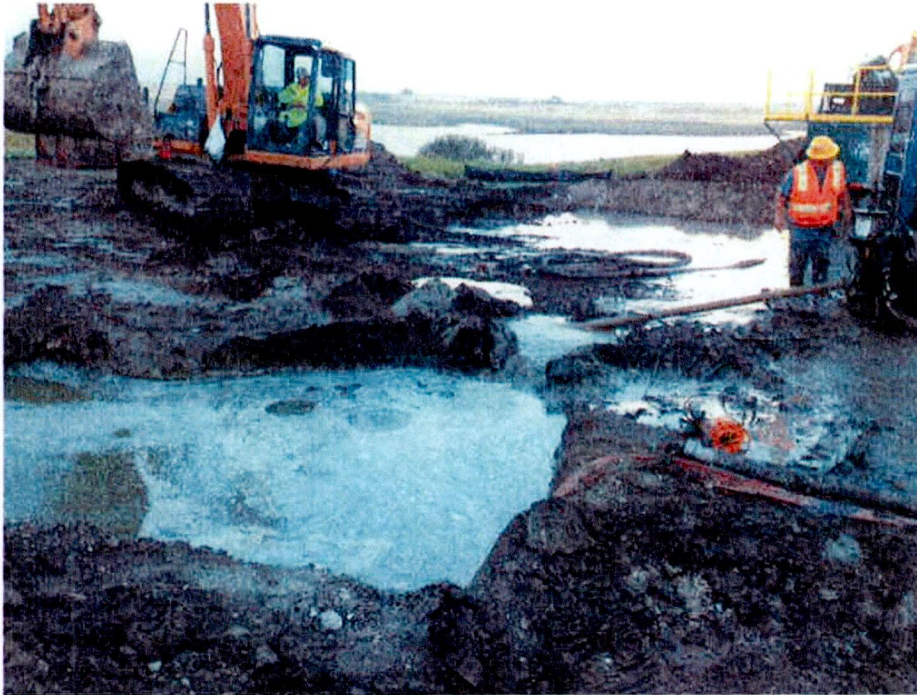
September 18, 2013 – Pulling pipe through bore hole under Cottonwood Lake.
