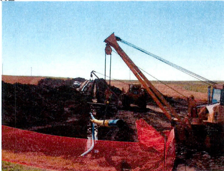
September 20, 2013 – Pipe installation at the boring location across 71 st Ave.
