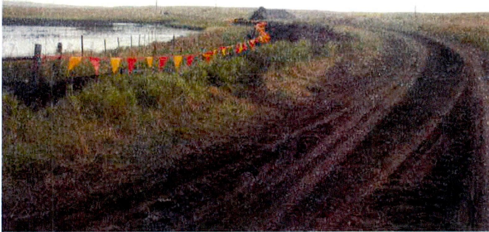
September 18, 2013 – Stripping activities near a flagged and silt fence protected wetland.
