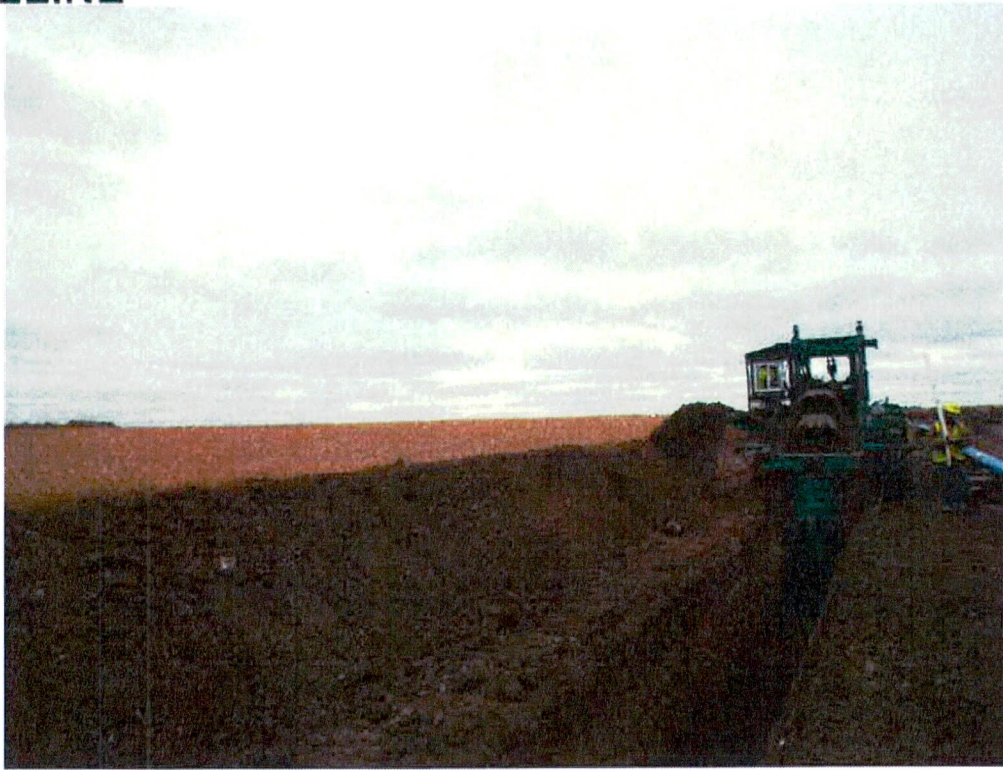
A trenching machine on the ROW.
