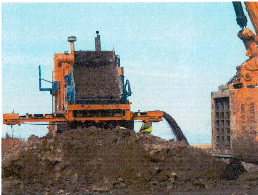
Remote operated backfill shaker, padding the pipe.
