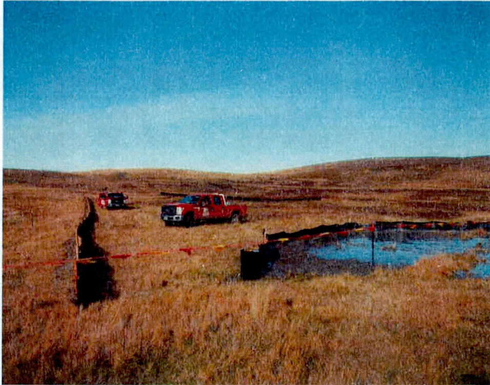
Silt fence contains drill mud.
