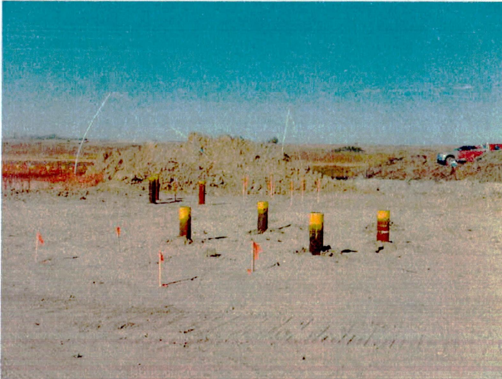
Block-valve pad location just south of 74 th Ave.
