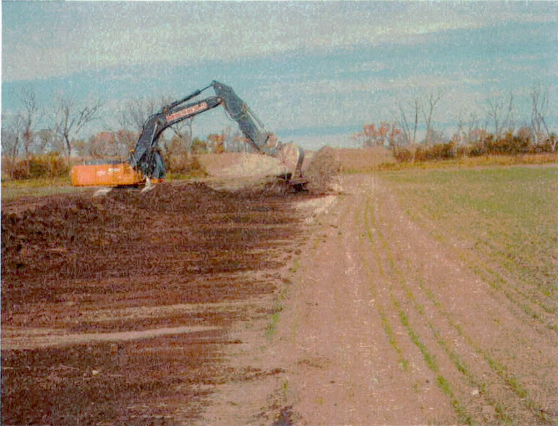
An excavator pulls topsoil back onto the ROW for spreading
