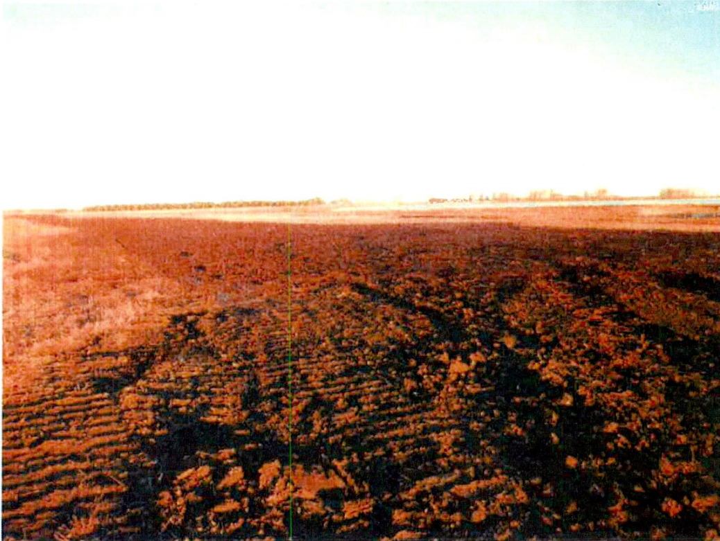
Re-graded ROW after topsoil placement.
