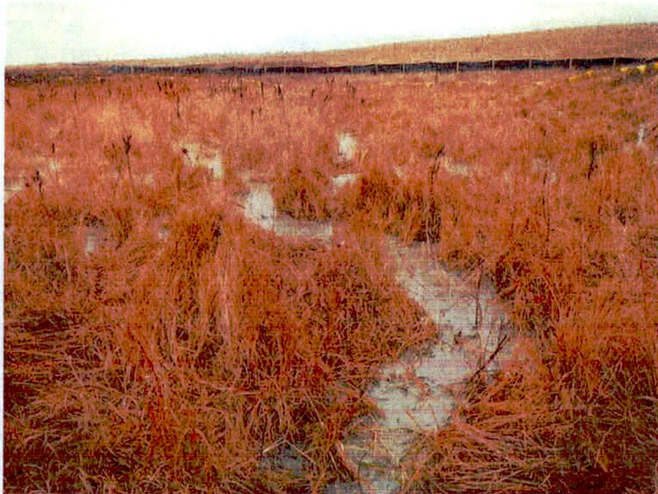
Straw wattles placed to divert water from cow paths onto pipeline corridor near MP68.06.
