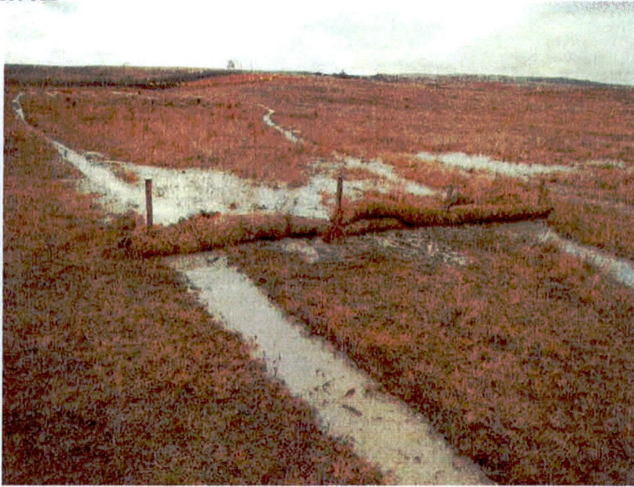
Straw wattles placed to divert water from cow paths onto pipeline corridor near MP68.06.
