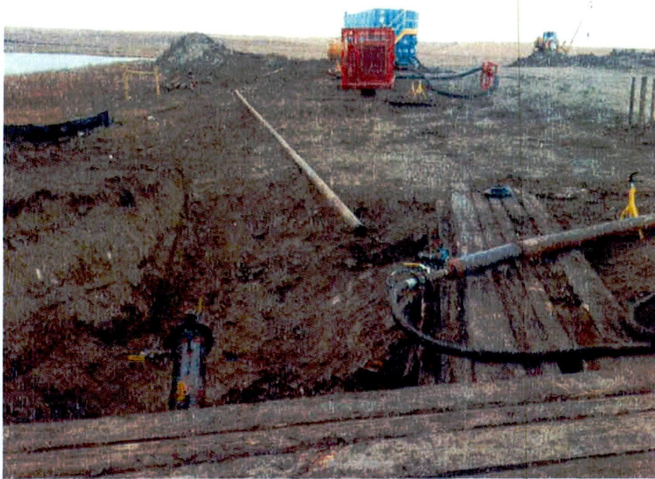
Pipeline preparation for hydrostatic testing with discharge pipe on the right.
