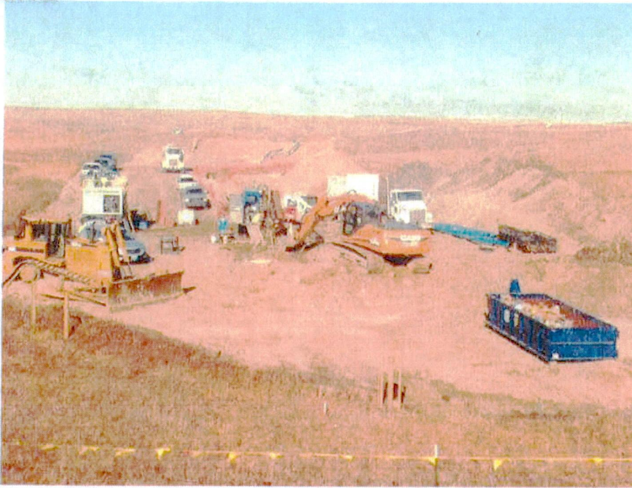
HDD boring activities at MP68.37.
