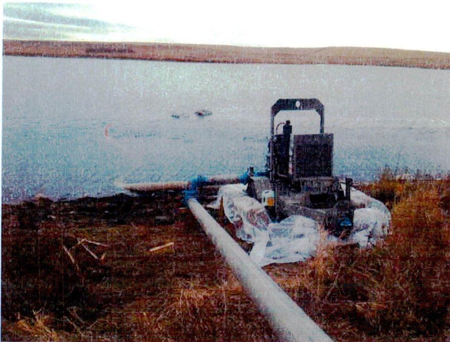
Pump setup for hydrostatic testing from Cottonwood Lake
