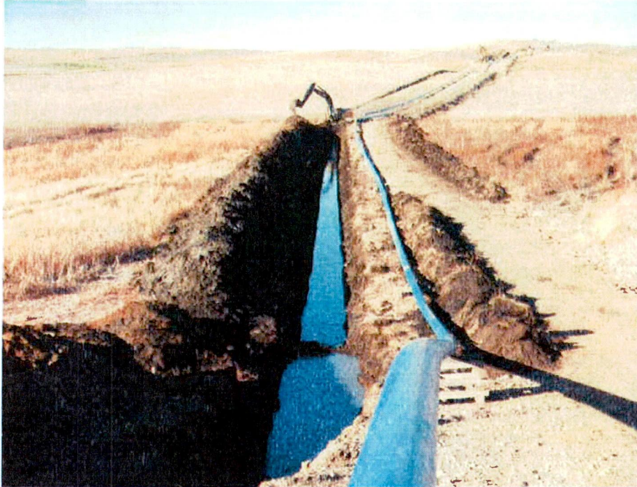
Trenching activities through wetland area at MP 65.65.
