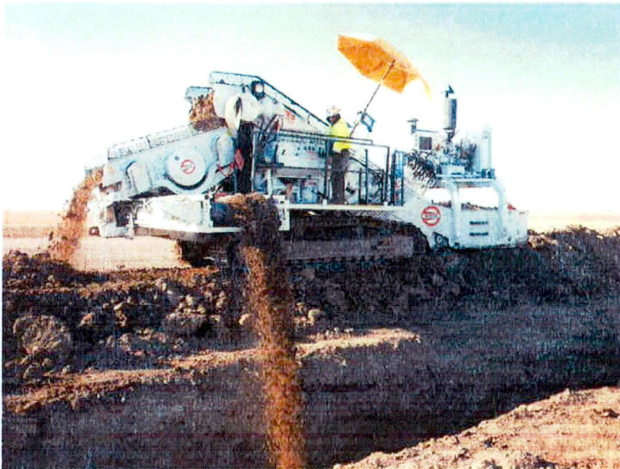
Padding/backfilling along ROW near MP 61.
