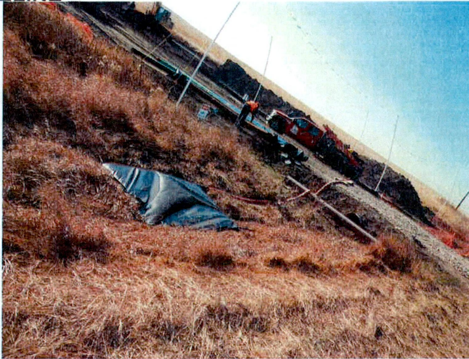
Stormwater dewatering activities from tie-in excavation along ROW.
