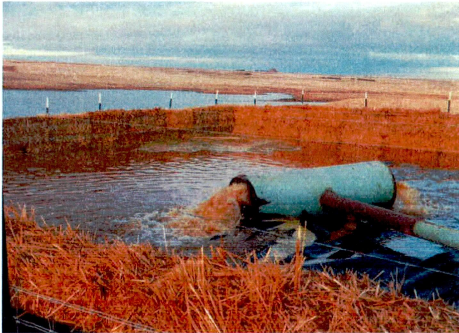
Hydrostatic testing discharge to the energy dissipation dewatering structure.
