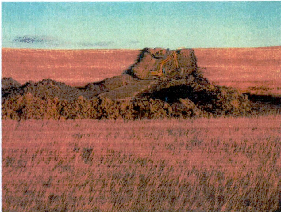
MP 77.30: Trench backfilling activities.
