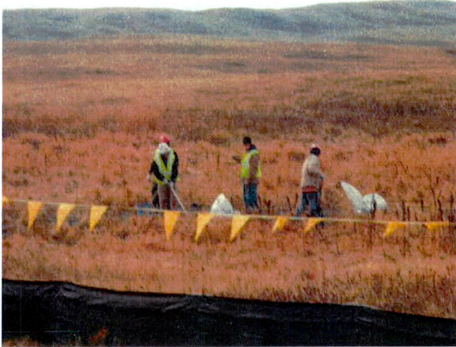
MP 68.02: Dry wetland cleanup activities in progress.
