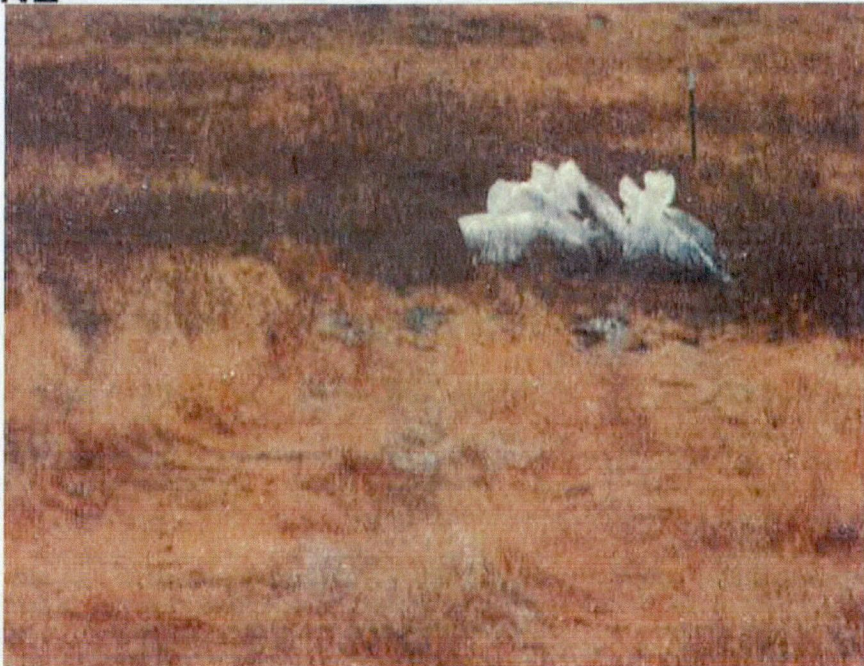
MP 68.01: Bagged drill mud staged for removal following removal from dry wetland.
