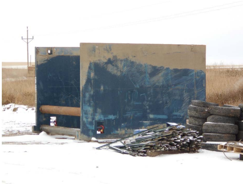
Photo 6 – An example of trench shoring used during construction of the project.
