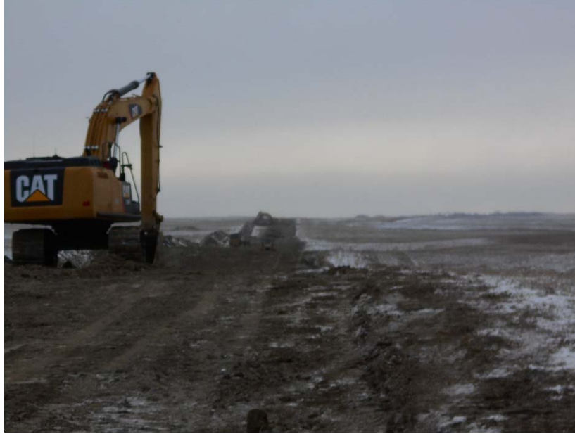
Photo 7 – Construction equipment replacing topsoil along the pipe route.
