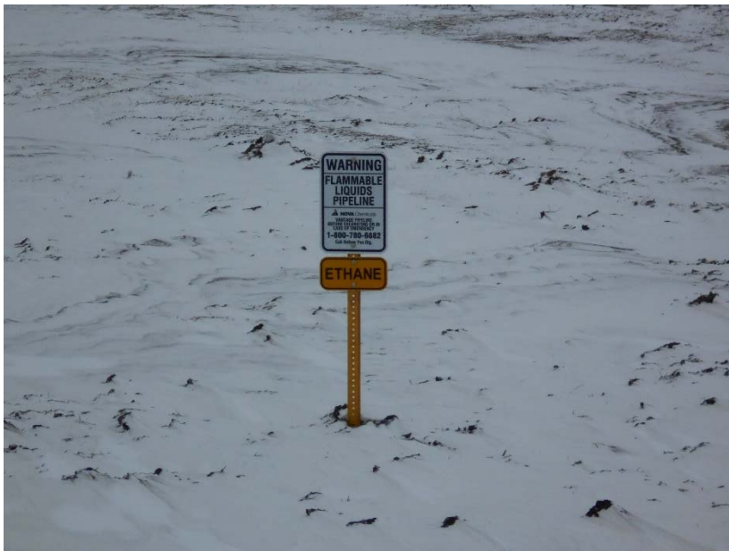
Photo 2 – Typical pipeline marker at road crossing.
