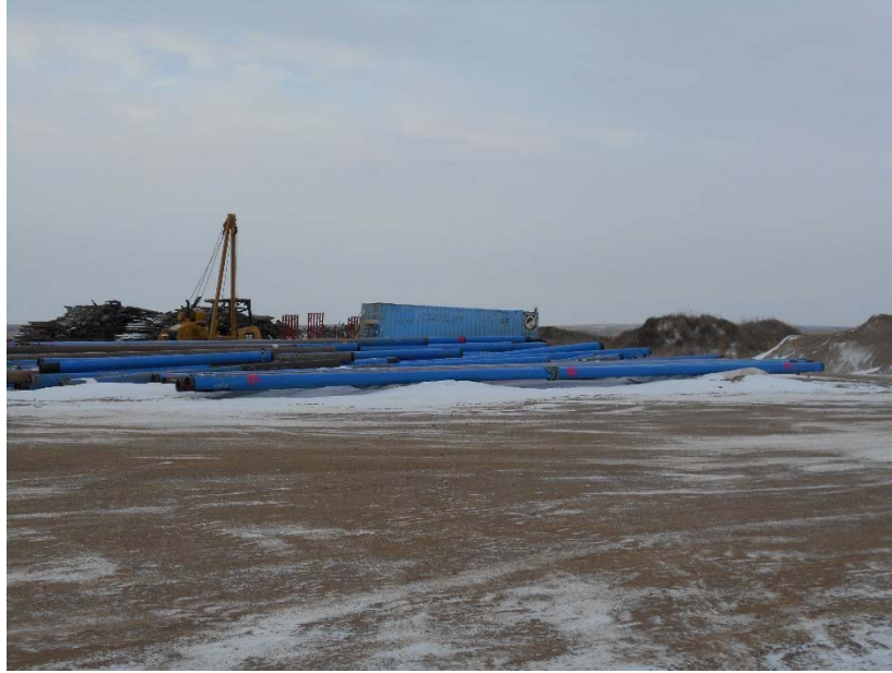
Photo 5 – Piping storage at contractors’ laydown area.
