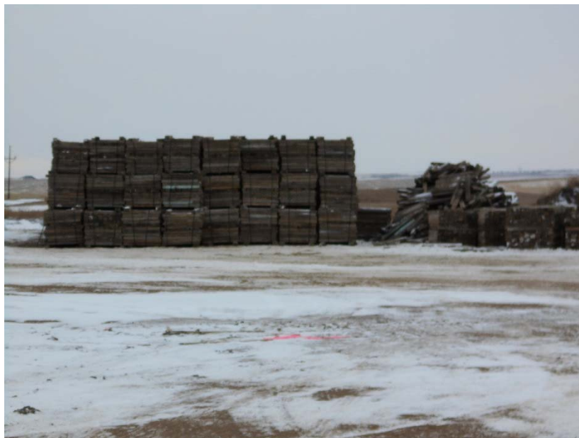
Photo 4 – Matting storage at contractor's laydown area.
