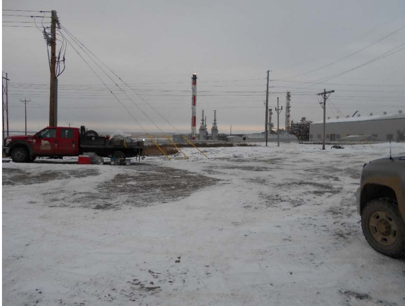
Photo 1 – Beginning of pipeline just north of the Tioga Hess Natural Gas Plant.
