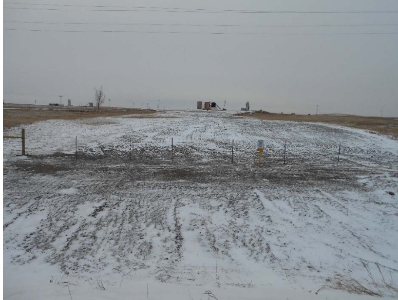
Photo 3 – Replaced fenced and pipeline marker.
