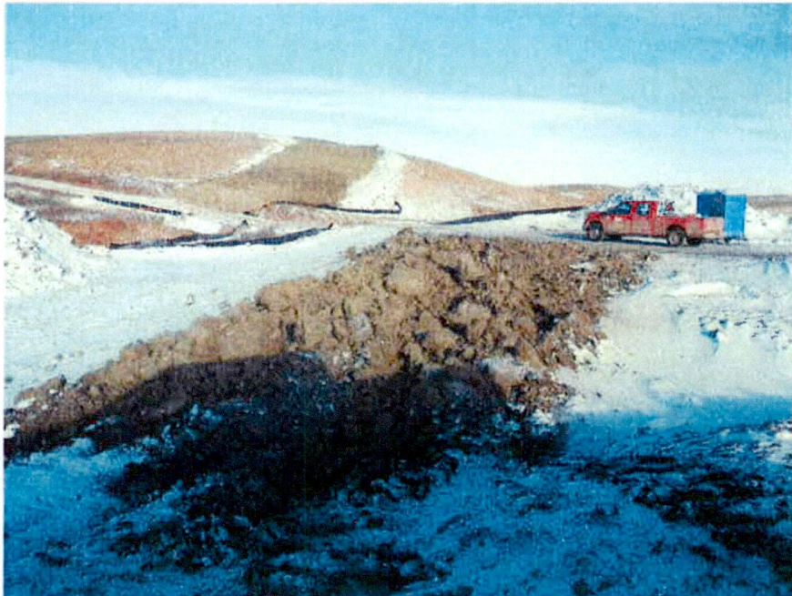
Frozen subsoil ripped with Dozer prior to spreading near MP 78.
