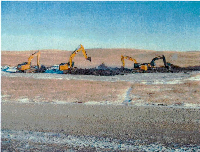
Topsoil spreading near MP77.5.
