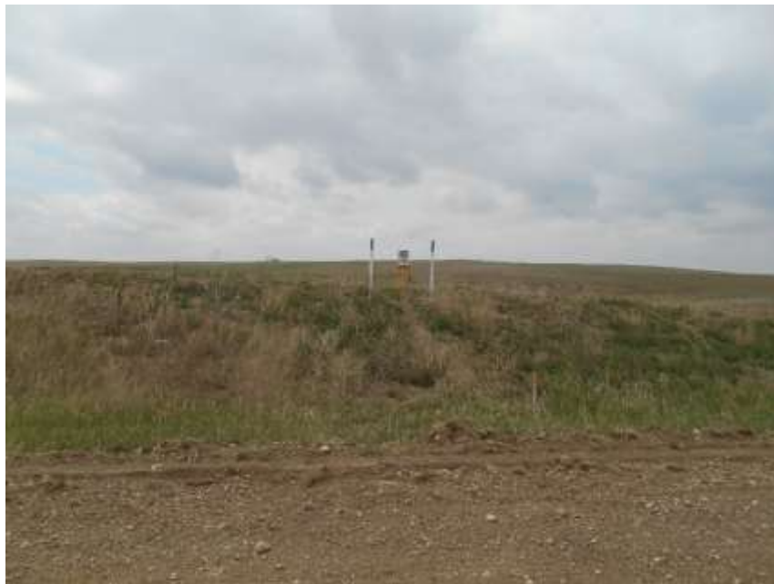
Photo 4 – 015: Typical pipeline markers at road crossing
