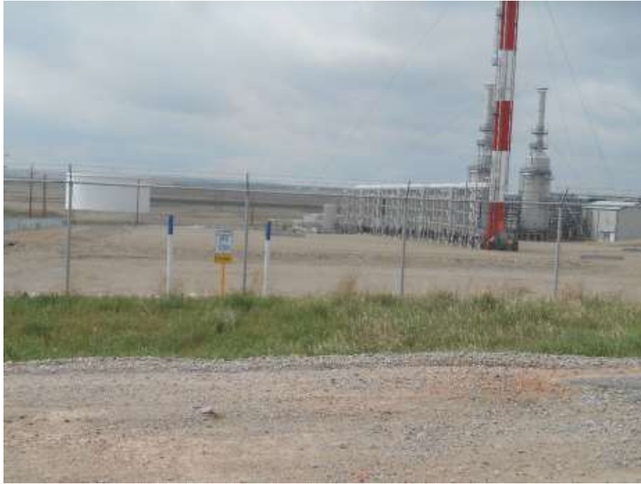
Photo 1 – 011: Hess Corporation’s Natural Gas processing plant
