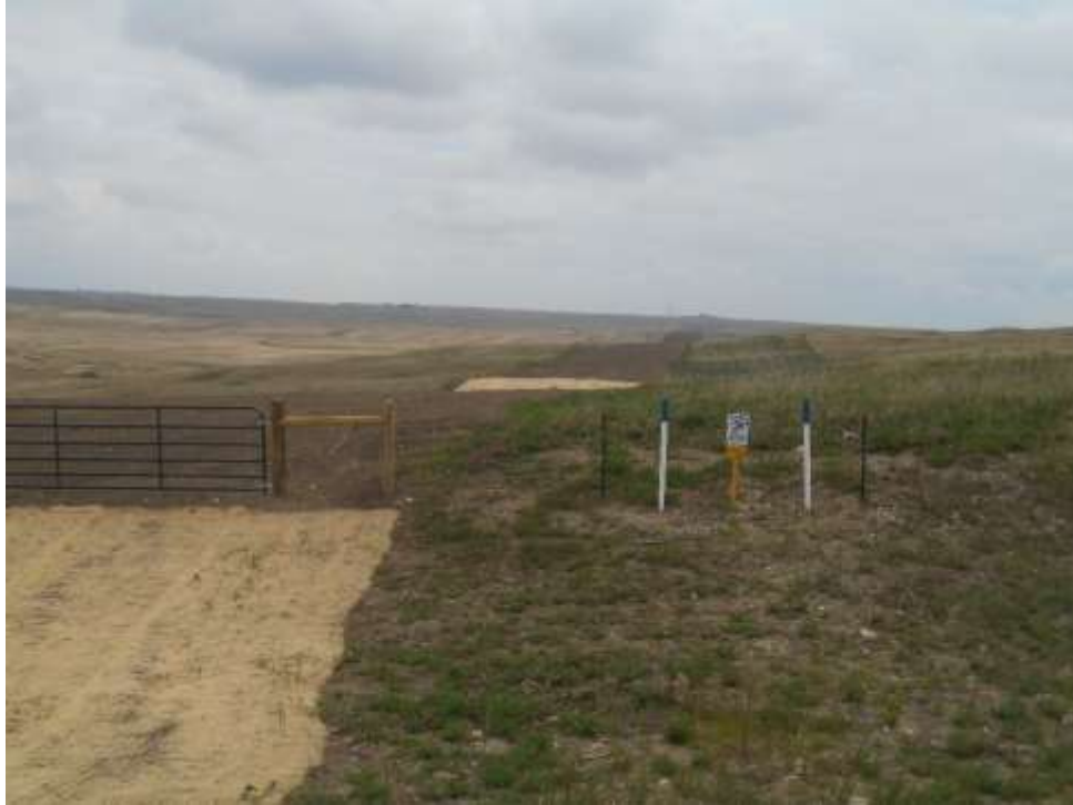
Photo 5 – 014: Shows the portion of the pipeline paralleled by another pipeline.
