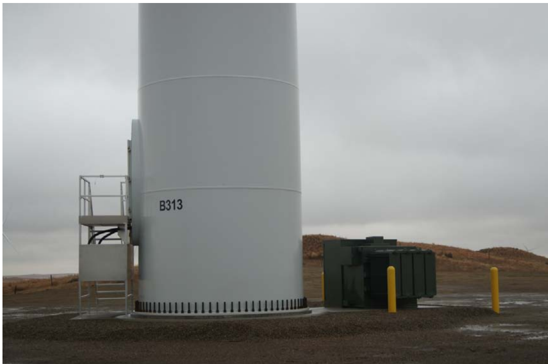
Turbine 313 located in sandstone rock
