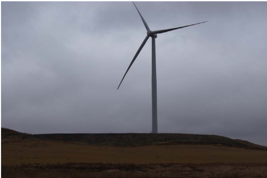
Turbine site 313 – sandstone rock area with final proper contouring
