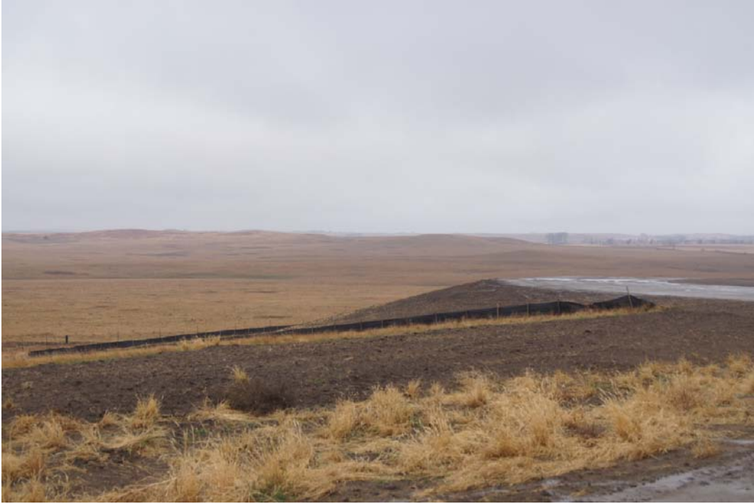
Erosion Control -Silt fencing
