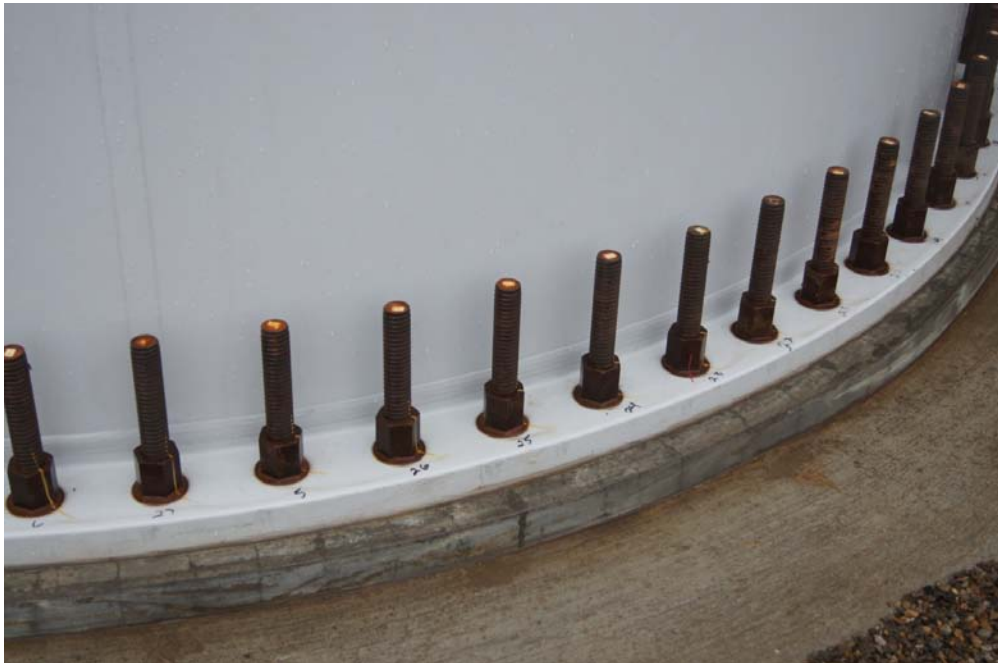
Turbine base bolting to foundation
