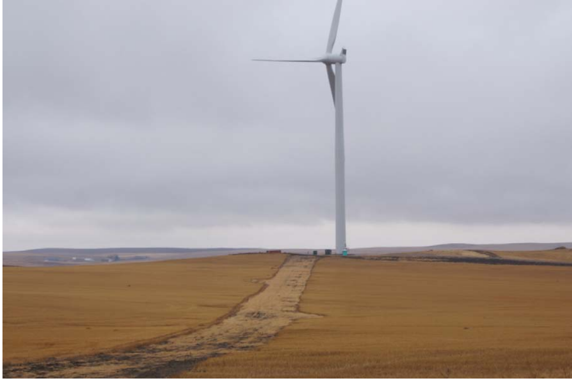
Crane path route restoration
