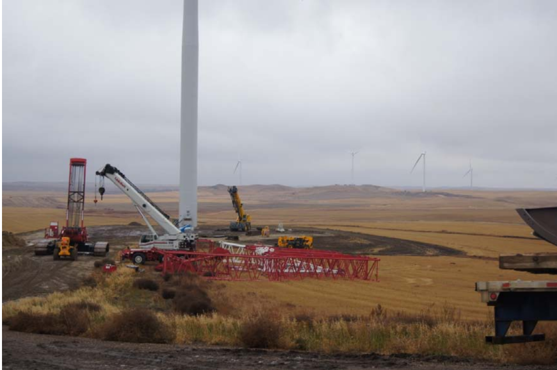
Construction crane tear down and removal
