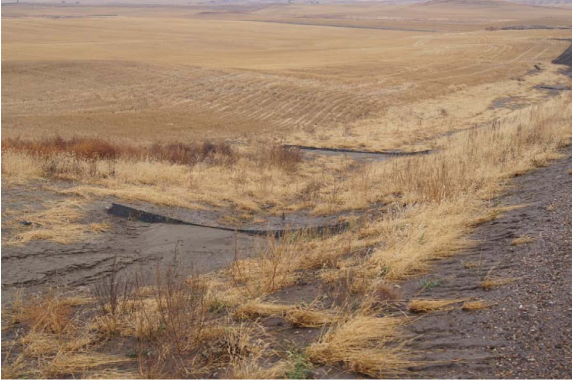
Erosion Control- Triangular containment fencing
