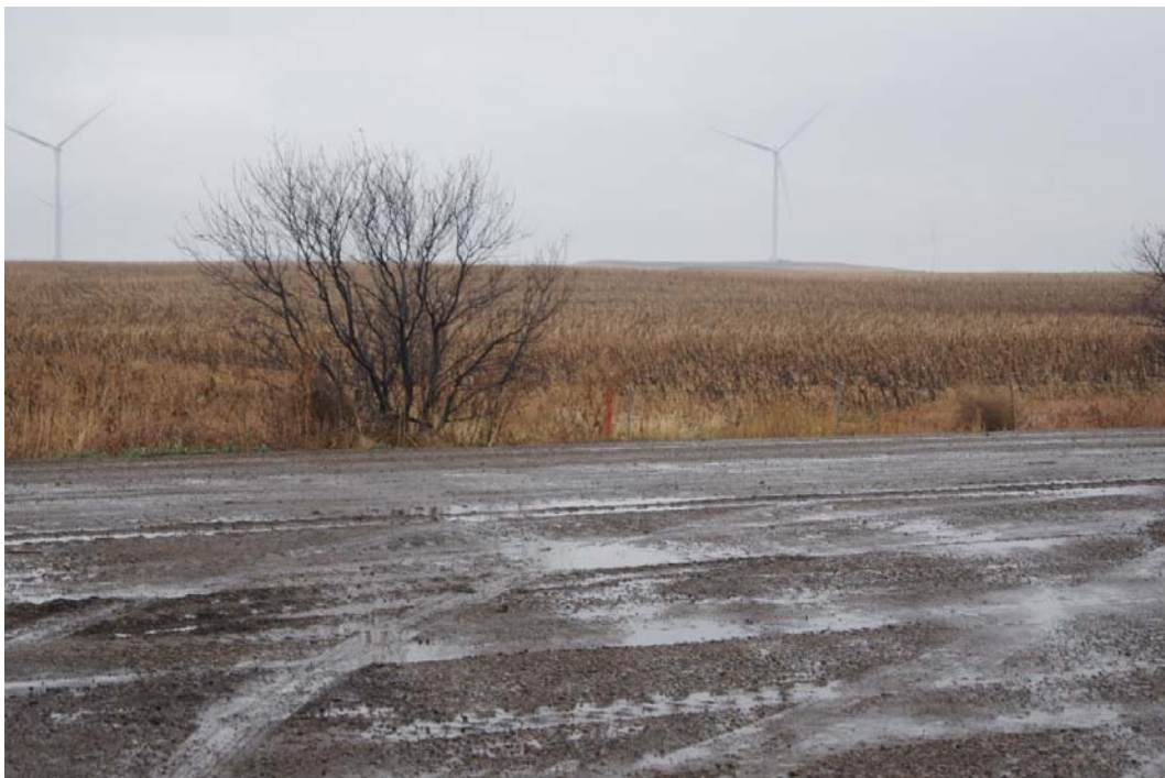
Line marker signs located at road crossings.
