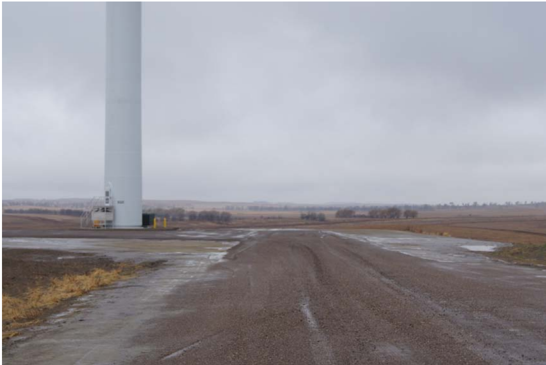
Turbine site 325 where final gate is to be installed across road
