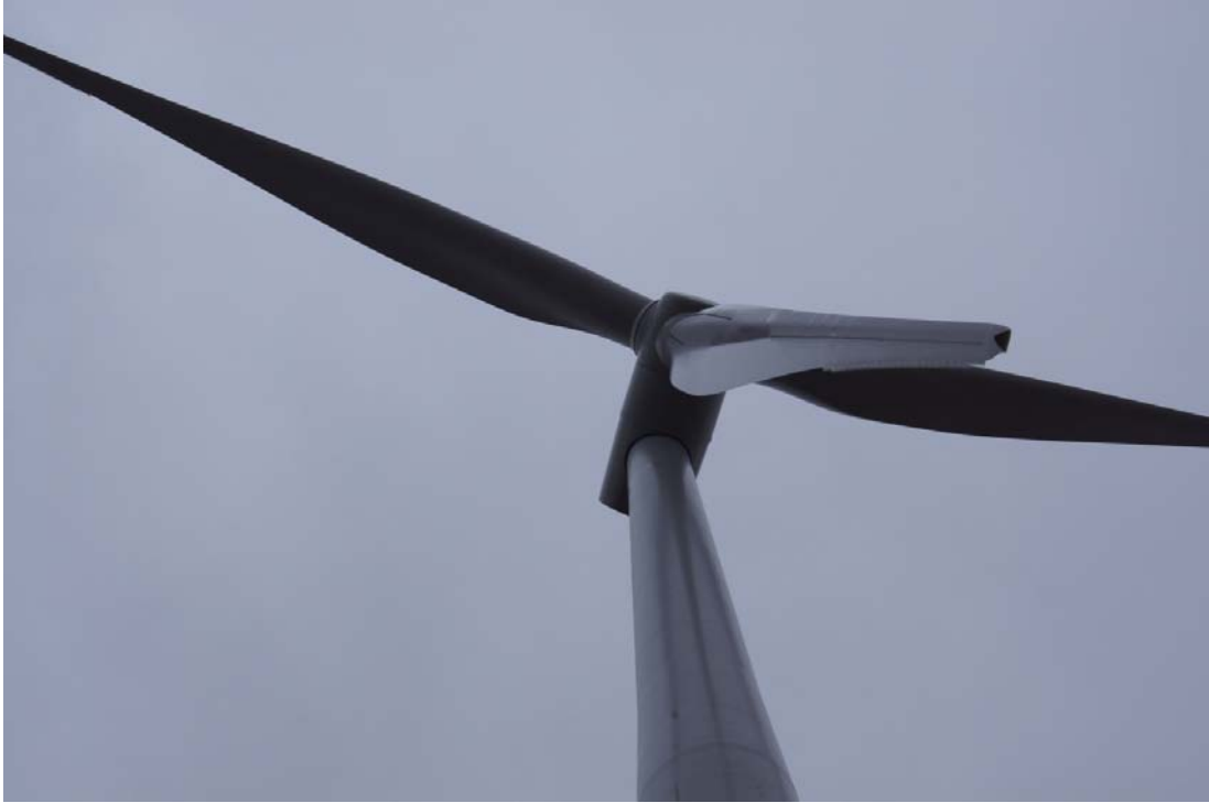
Siemens 3.0 MW turbine model SWT-3.0-101
