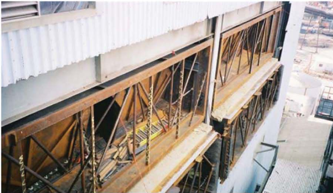
Figure 3-3. Boiler Building Wall Openings
