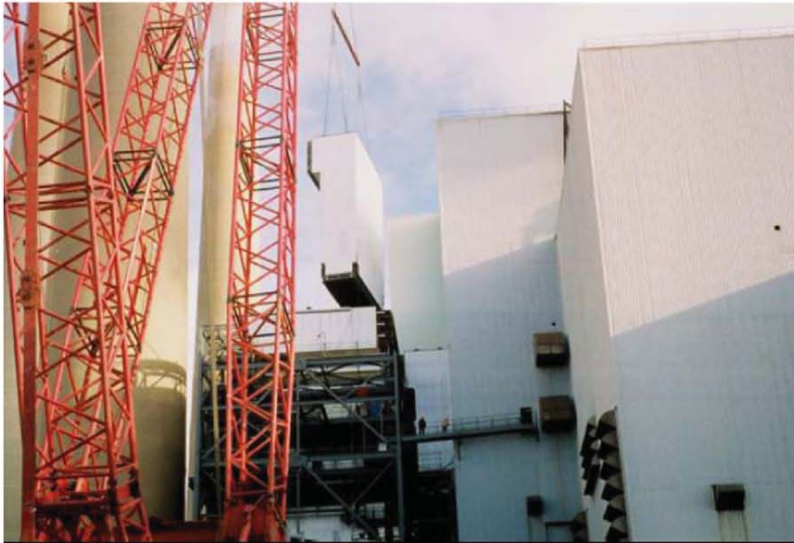
Figure 3-4. Example of SCR Inlet Duct Installation During Plant Outage
