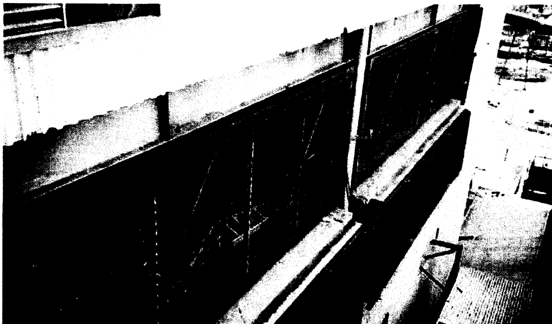
Figure 3-3. Boiler Building Wall Openings
