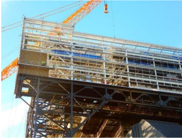
2014-10-07 Siding on SCR
