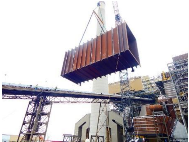
2014-11-03 G28 duct lift
