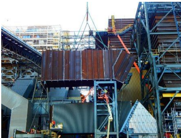
2014-10-07 G26 ID fan 1A discharge ductwork lift
