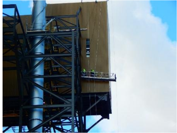
2014-12-09 Siding work continues
