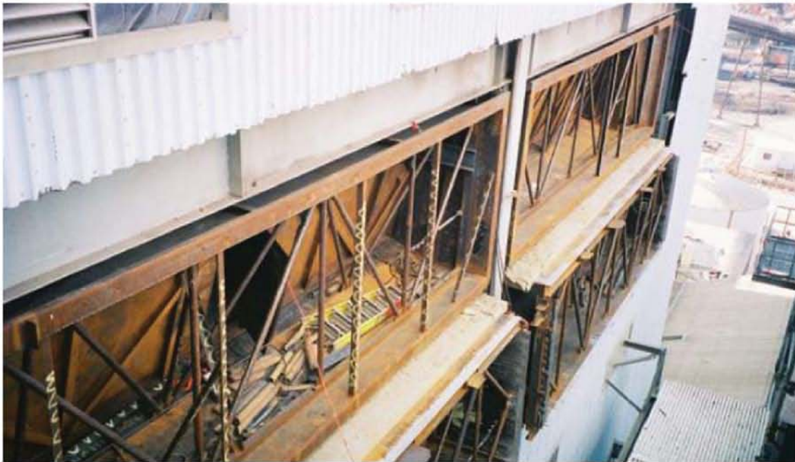
Figure 3-3. Boiler Building Wall Openings
