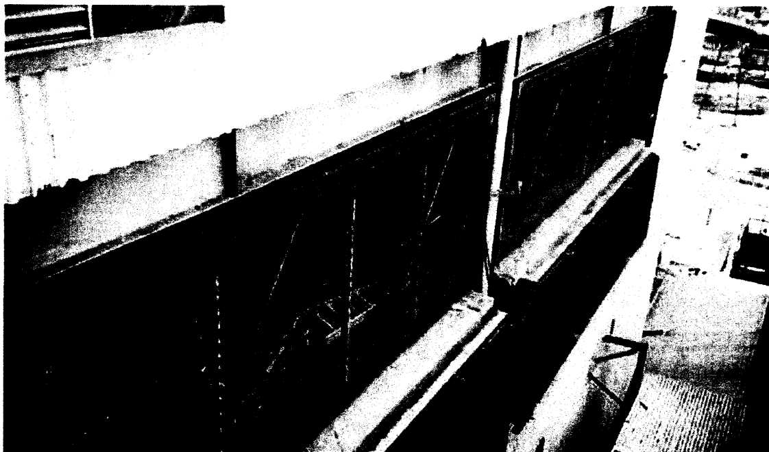
Figure 3-3. Boiler Building Wall Openings
