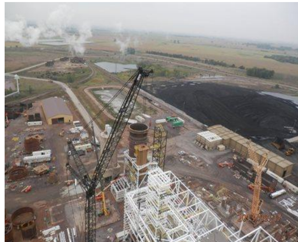
09-17-13 Site overview to south
