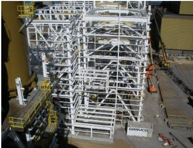
09-14-13 Absorber & baghouse structural steel erection
