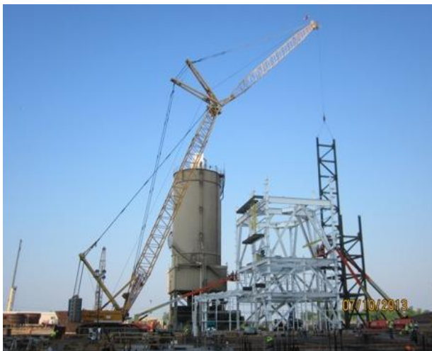
07-10-13 WA & PI stair tower erection
