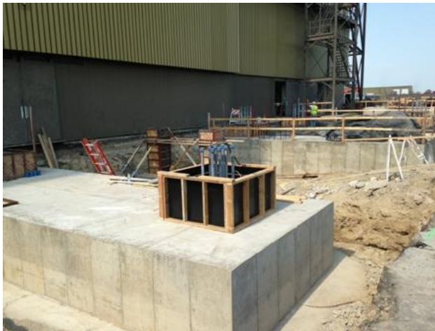
08-23-13 North SCR tower foundation
