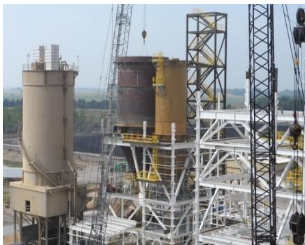
09-09-13 Waste ash & pebble lime silo erection
