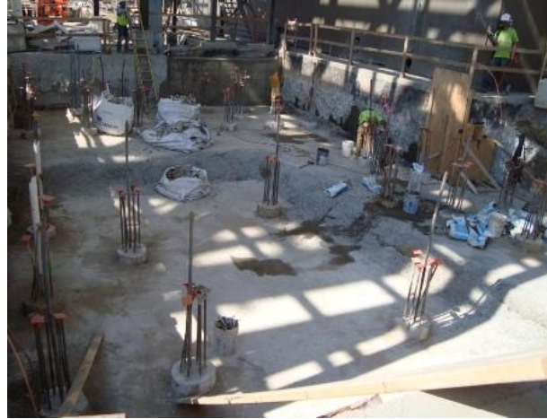
09-07-13 Prepping South SCR piling
