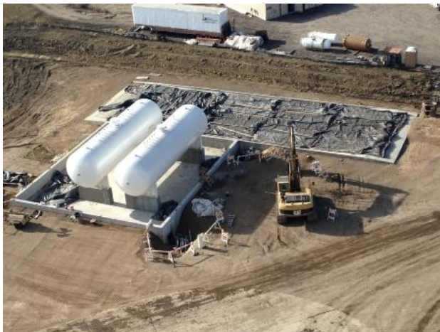
11-20 Ammonia tanks set & unloading slab poured
