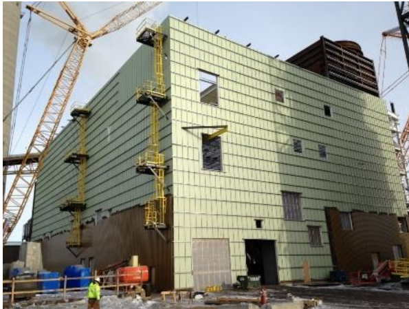
12-11 Insulation & siding on baghouse ongoing
