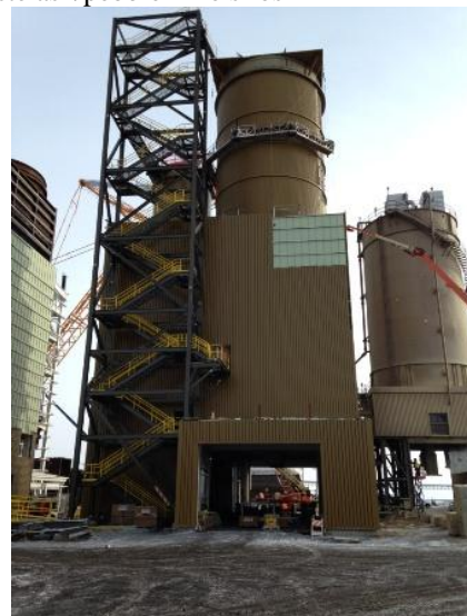
12-11 Siding work almost finished WA/PL
