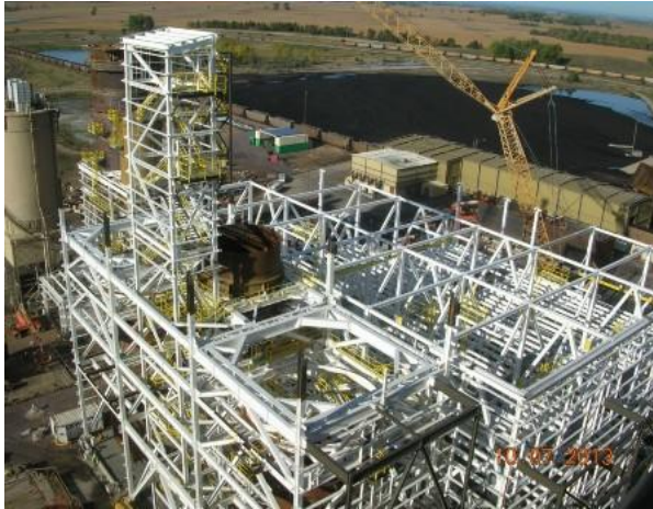
10-07 CFB & baghouse structural steel erection
