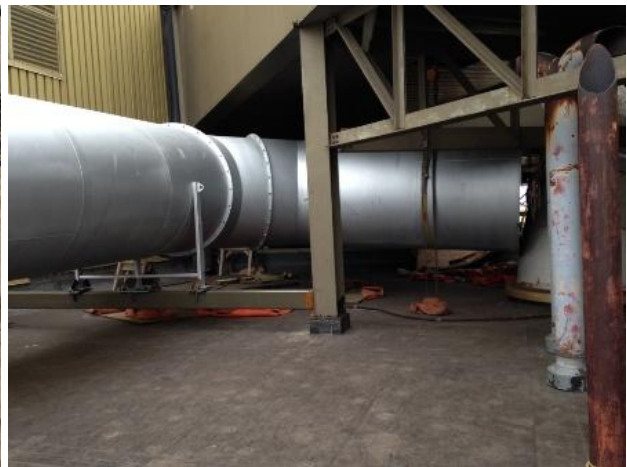
11-25 Setting aux boiler stack horizontal section
