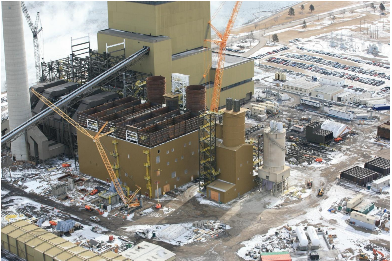
03-28-2014 Aerial View Taken
