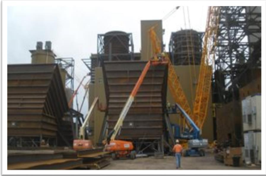
2014-06-16 Ground assembly CFB outlet ducts
