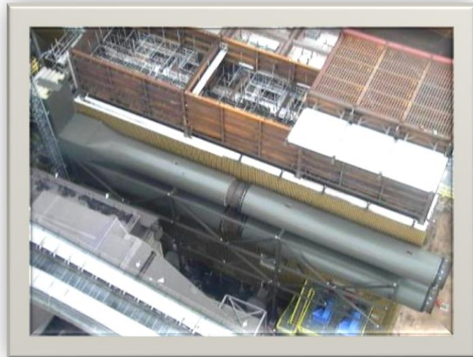
2014-06-05 Recirculation ducts in place
