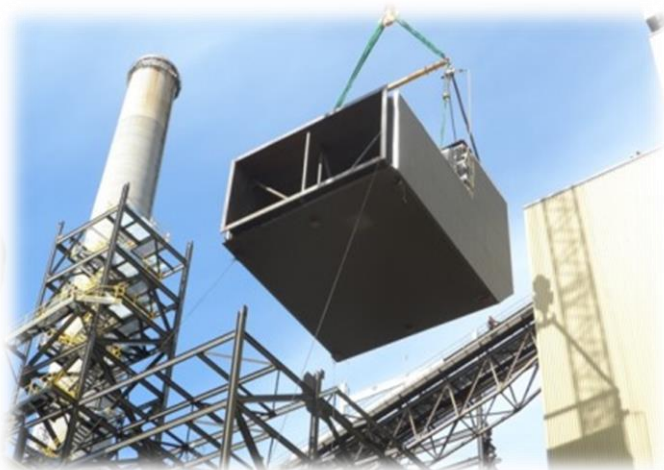
2014-04-08 G5B duct lift
