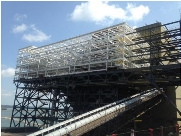
08-20 SCR grating install
