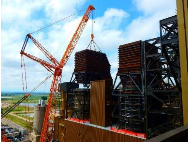
08-15 Setting train 2 outlet transition elbow, 1 set
