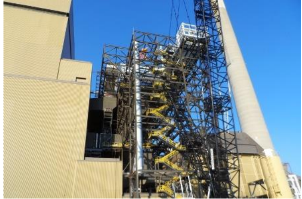
07-08 North SCR tower
