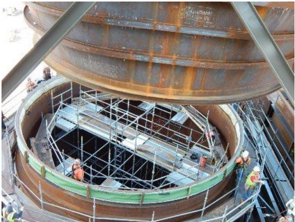
08-13 Setting train 1 outlet elbow
