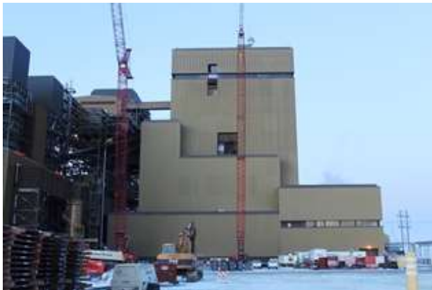
02-25 B&W openings south side of building
