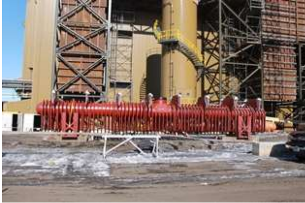
03-05 Reheat outlet header unloaded awaiting install
