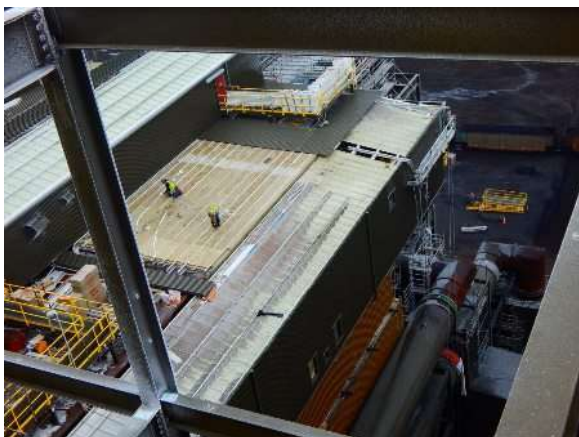
02-09 Insulating baghouse north
