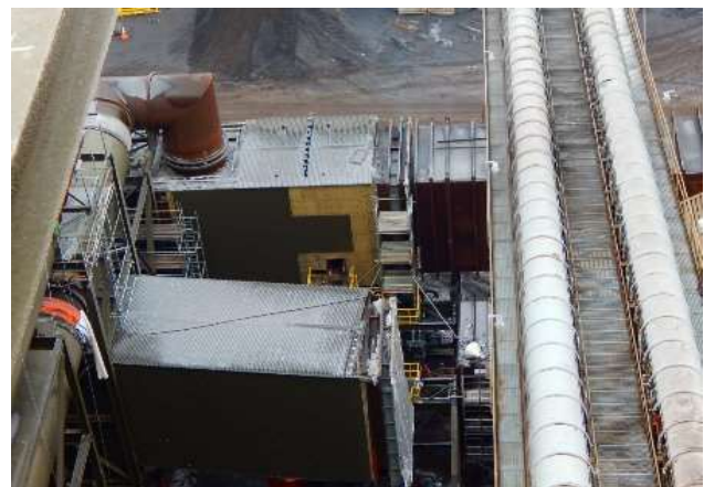
02-09 Insulating ID fan to chimney ductwork
