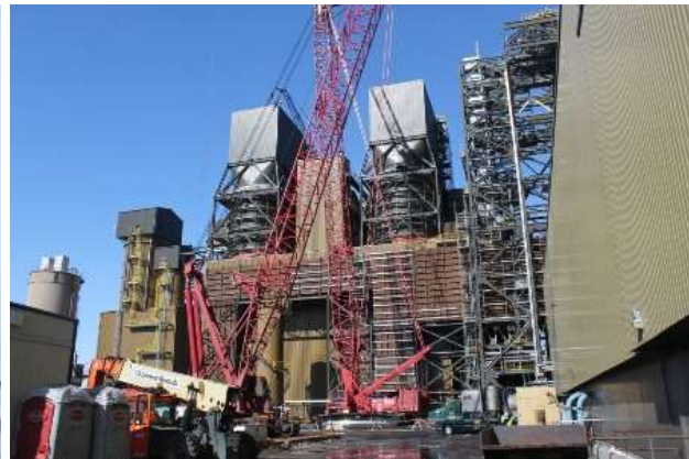
03-05 B&W cranes south side
