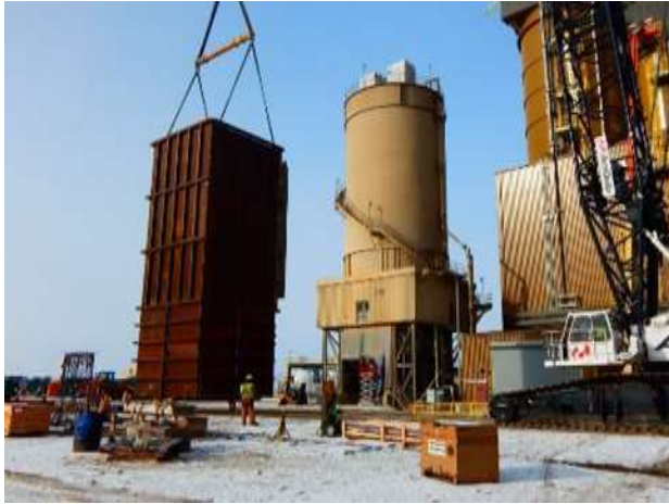
01-14 Setting section 7 CFB inlet ductwork
