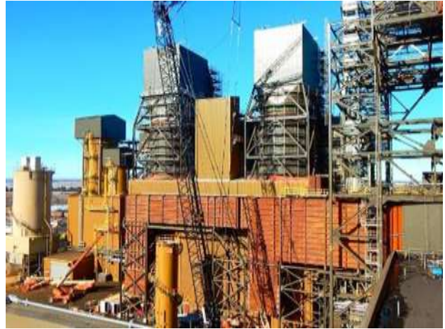
01-26 Final CFB inlet ductwork sections & activated carbon injection silo set
