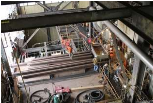
03-12 14th floor reheat header outlet removal
