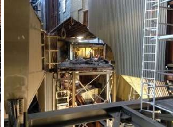
03-09 Air heater outlet duct demo
