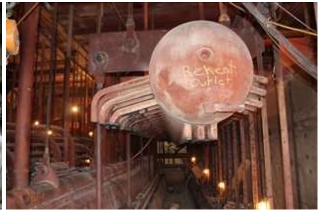
03-12 14th floor reheat header outlet removal
