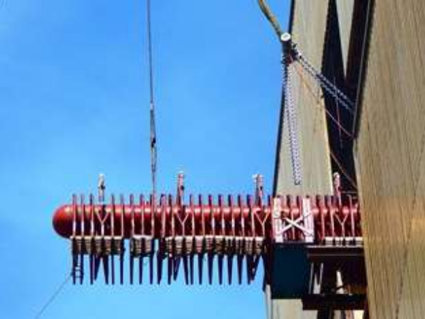
04-02 Reheat header removal
