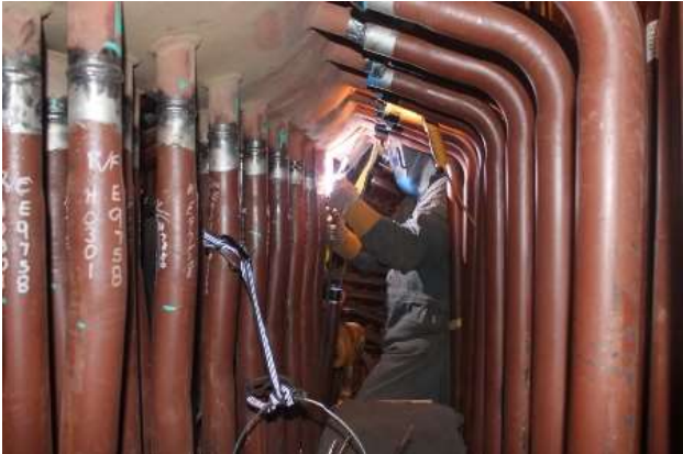
04-01 Welding in reheater inlets
