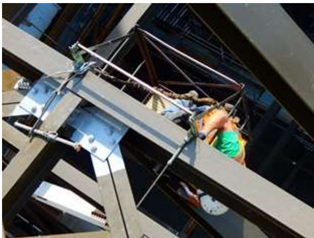
06-10 Painting structural steel
