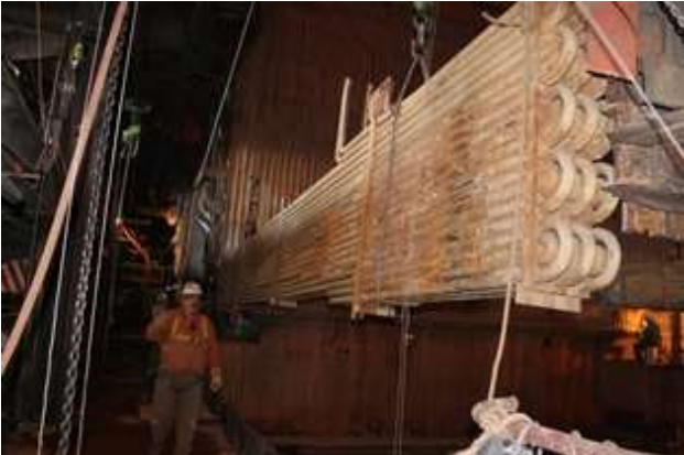
04-01 Removing primary module
