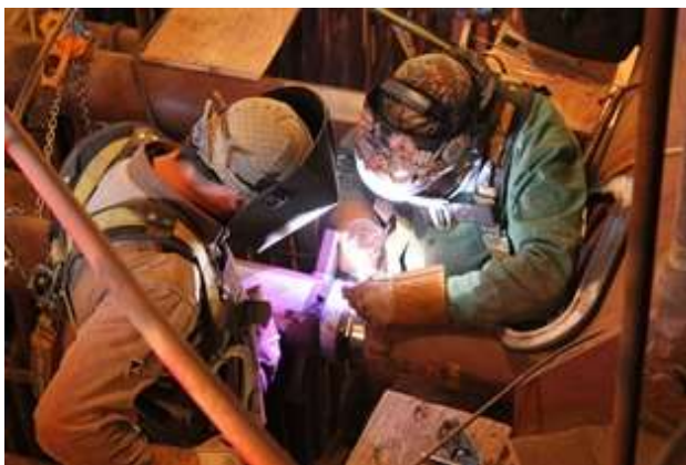
04-28 Welding inlet modules in secondary superheat
