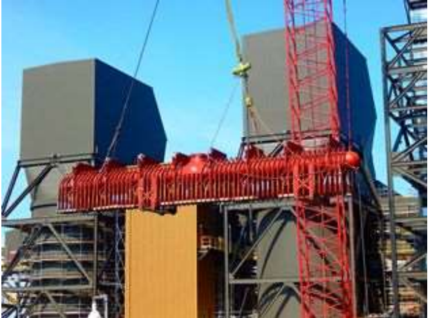
04-04 New reheat header lift
