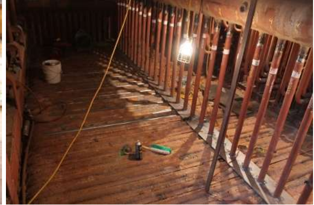
05-14 Install refractory on penthouse floor
