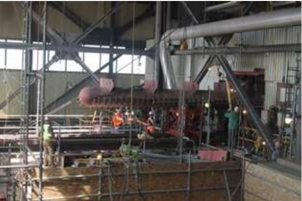
04-02 Reheat header removal
