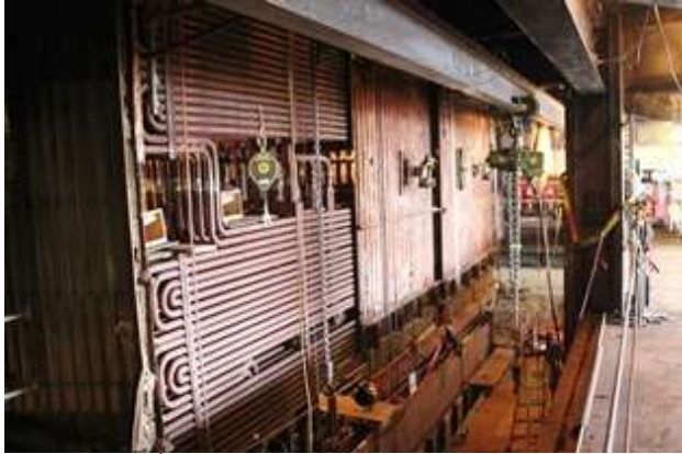
05-07 10 th floor convection pass sidewall install
