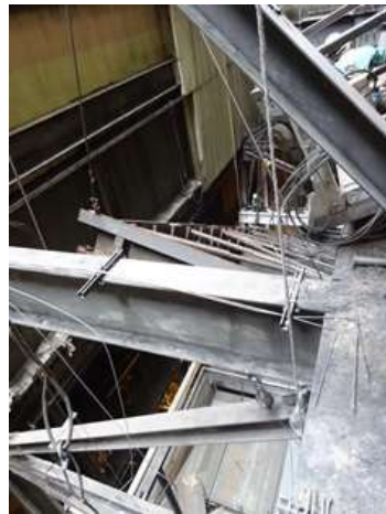
04-15 Progression of G6A duct lift
