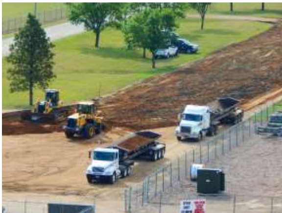
07-07-15 Reclaim of parking lots begins
