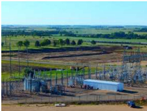
07-29 Reclaim of main laydown area
