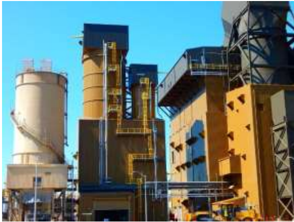
08-20 Close-up WA/PL (old ash silo will be removed)
