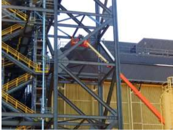
07-07-15 SCR (painter on JLG doing touchup painting)
