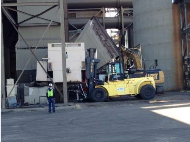
2015-10-07 Veit mobilized and beginning Demo work – ID Fan motors being removed
