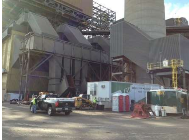
2015-10-07 Veit mobilized and beginning Demo work – ID Fan motors being removed
