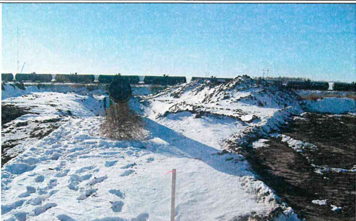
20-inch pipe, installed under railroad tracks.
