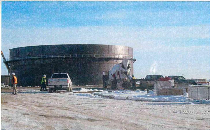
Partially complete tank, looking east.
