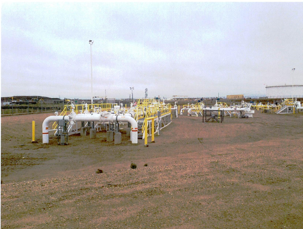
Photo 4: Restoration of disturbed construction area.
