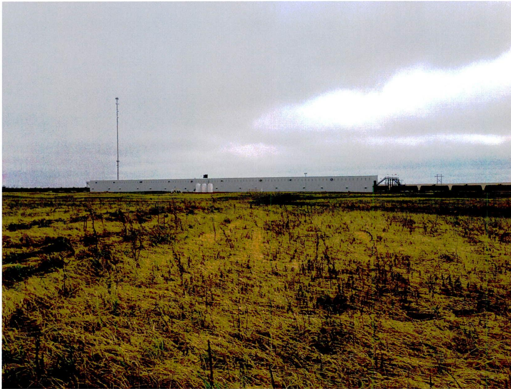
Photo 1: View of successful revegetation along the pipeline right-of-way.
