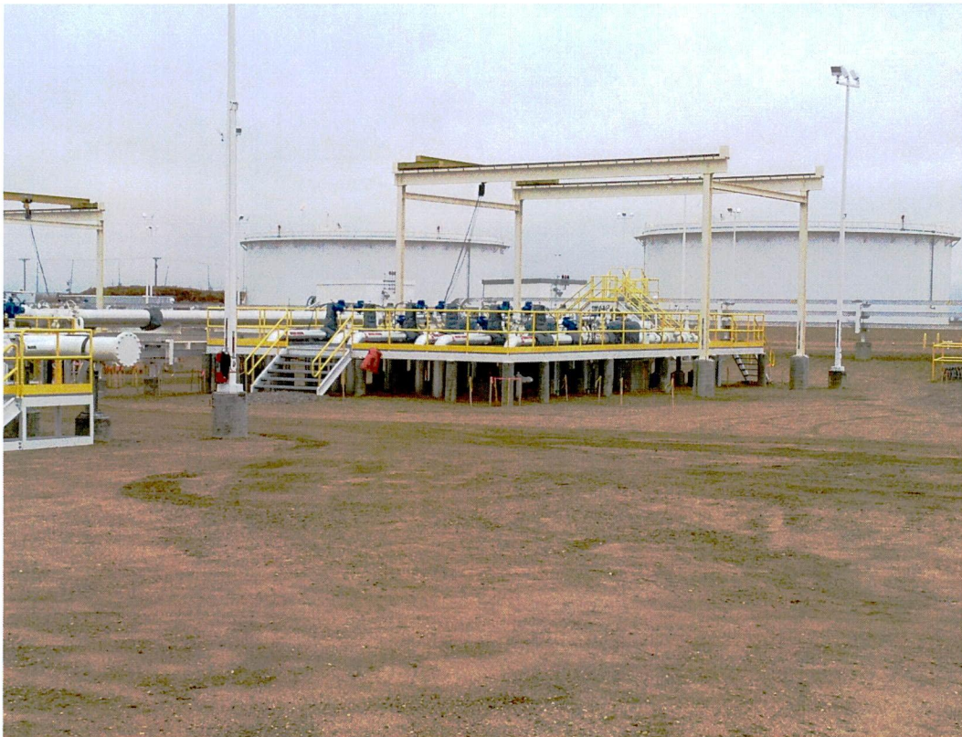
Photo 5: Restoration of disturbed construction area.
