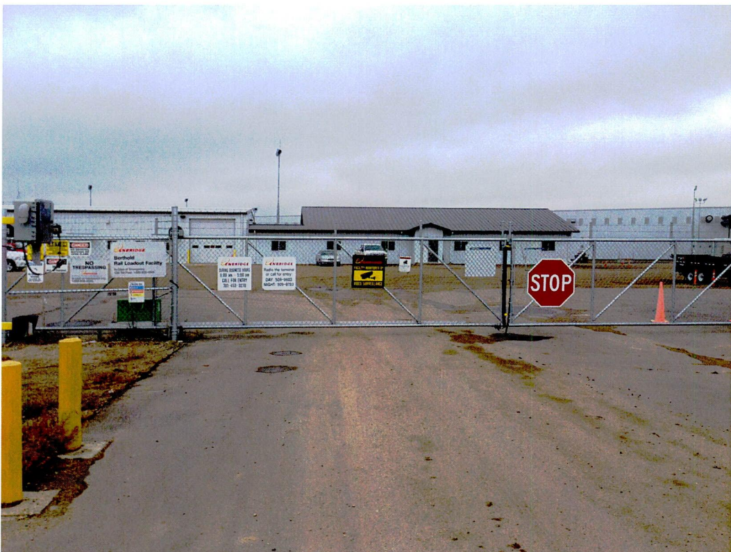
Photo 2: Controlled access to Enbridge facilities.
