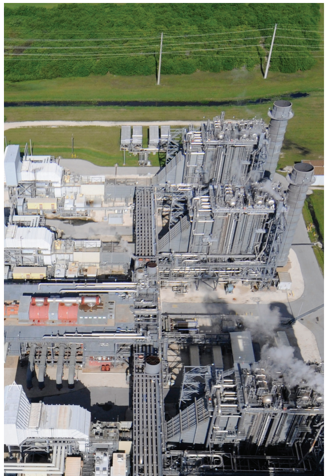
Florida Power & Light employs clean, highly efficient combined-cycle technology to reduce air emissions and fuel costs.
