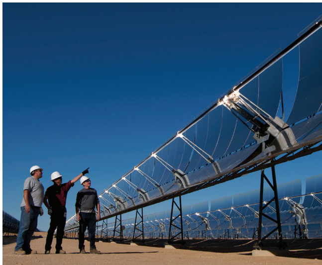
More than 900,000 mirrors concentrate heat from the sun at the Solar Electric Generating Systems operated by NextEra Energy in California's Mojave Desert.
