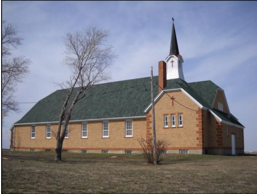
Photograph 12 (Northwest): A view of St. Vincent Catholic Church from the church lawn southeast of the building.
