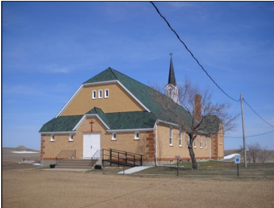
Photograph 11 (Northeast): A view of St. Vincent Catholic Church from the church parking lot.
