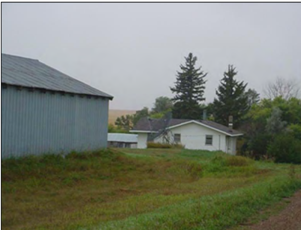
Photograph 2 (South): A view a metal outbuilding east of the house at 32MOx541 from 35th Street. This photograph was taken 8/28/2009 by Swenson, Hagen & Company.
