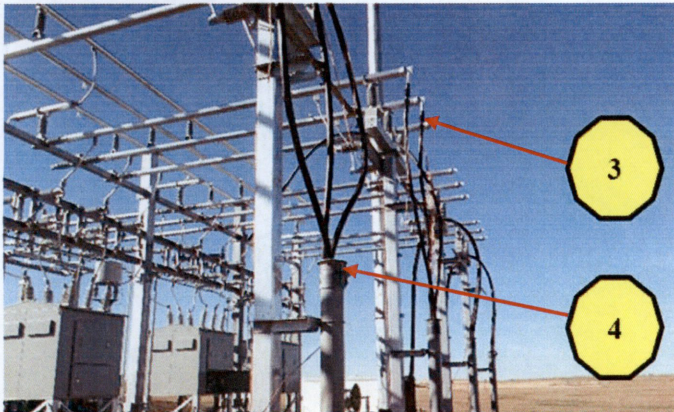
Circuit 4 that was to be tested, circuit 3 that the substation crew were working on
