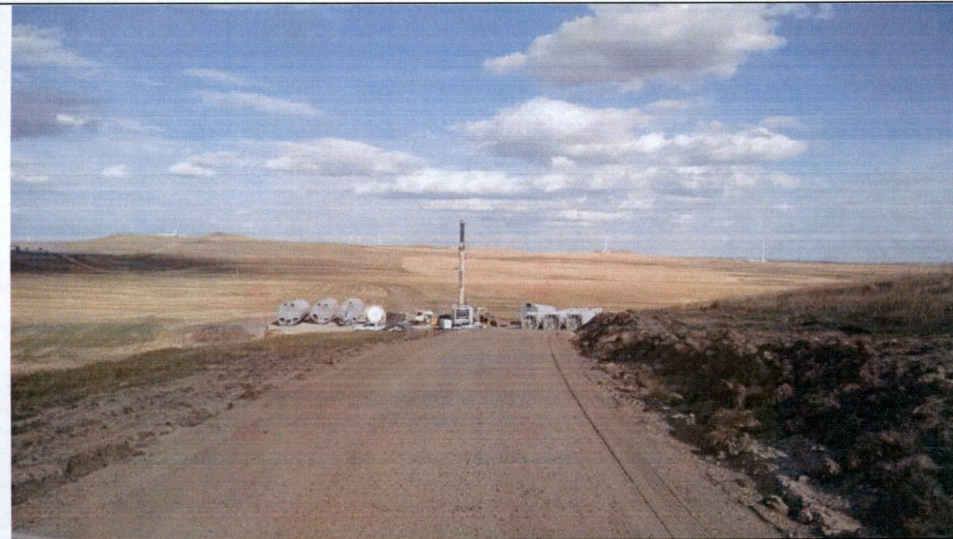
Photo 10: Preparing to assemble tower at Turbine 27.
