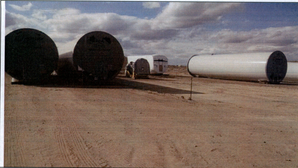
Photo 7: Tower sections and nacelle staged on the pad for Turbine 15.
