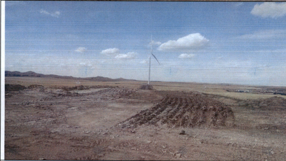
Photo 2: Topsoil respreads on reclaimed right-of-way.
