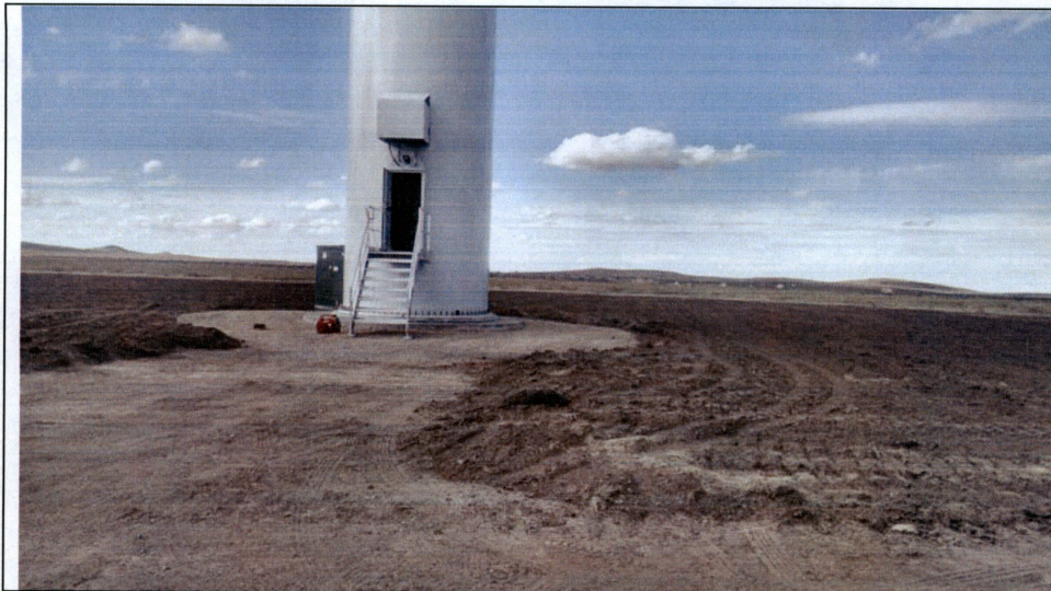
Photo 1: Completed turbine site, awaiting final preparation of seed bed.
