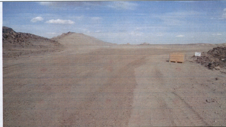
Photo 4: Foundation and subsurface grading complete at Turbine 13.
