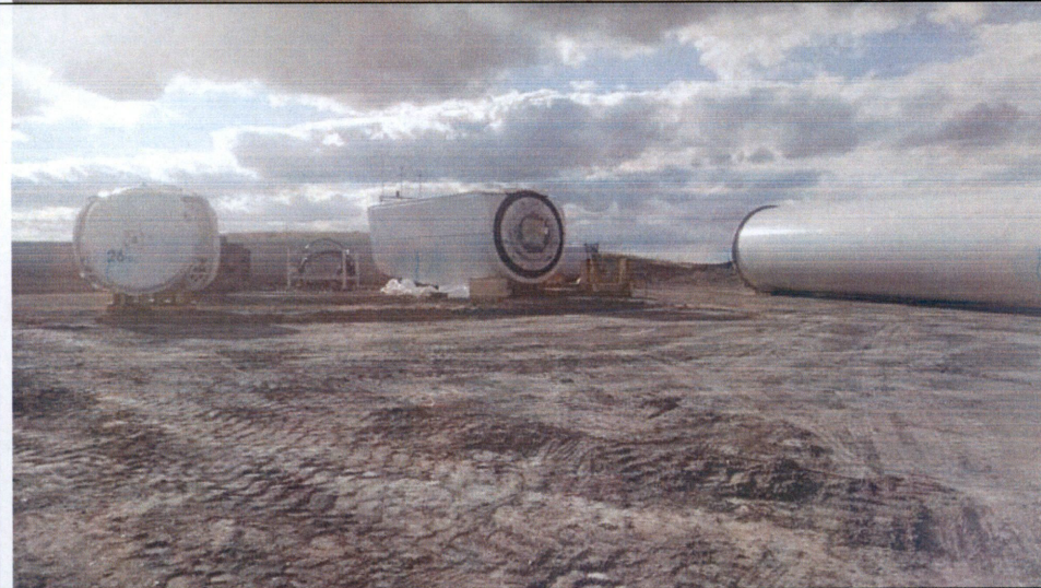
Photo 11: Tower sections and nacelle staged on the pad for Turbine 26.
