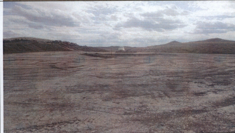
Photo 5: Completed subsurface grading at Pad for Turbine 9.
