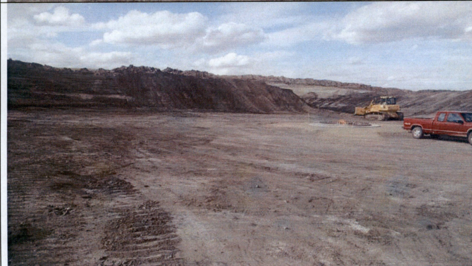
Photo 6: Re- spreading topsoil over excavated slope near Turbine 8.
