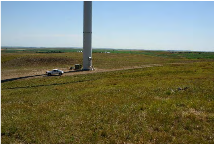
Photo 9: Tower 40 (facing East).
