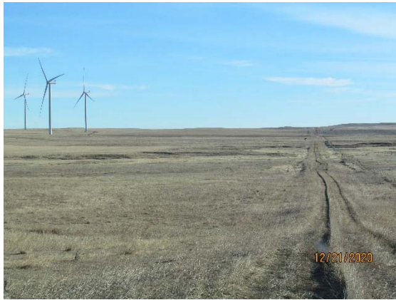
Photo 3: Section line (3 rd Avenue NE) roadway rutting, facing east.
