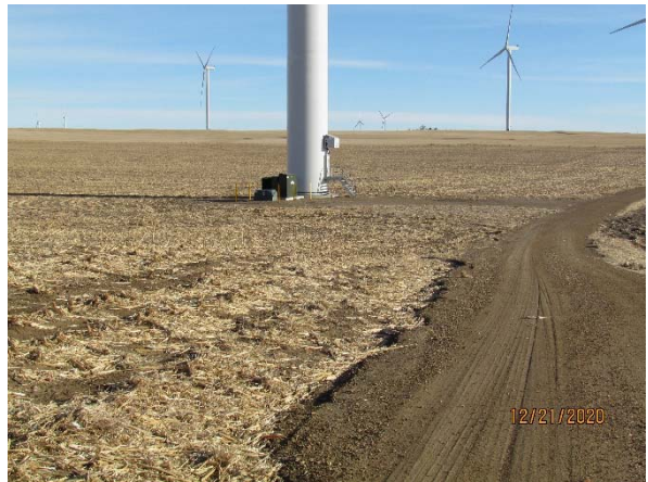
Photo 10: Minor erosion on Turbine 2, 3, 4, 5 access road, facing east.
