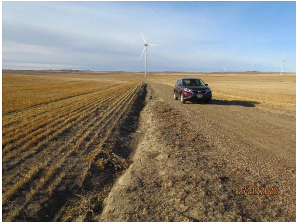
Photo 19: Erosion near Turbine 3, south side of access road, facing west.
