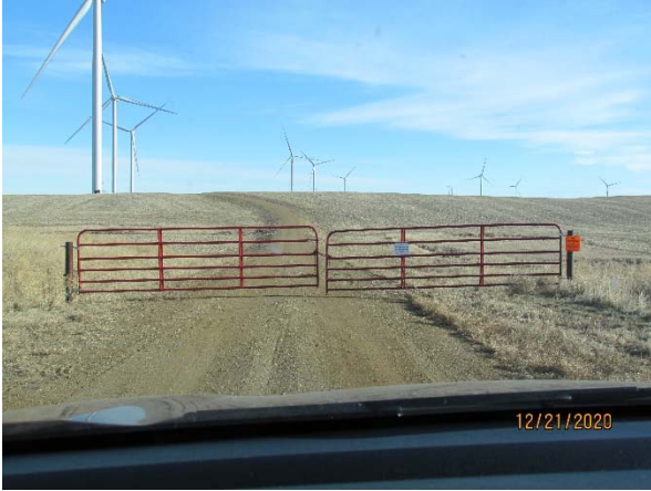
Photo 37: Turbine 14-16 access road.
