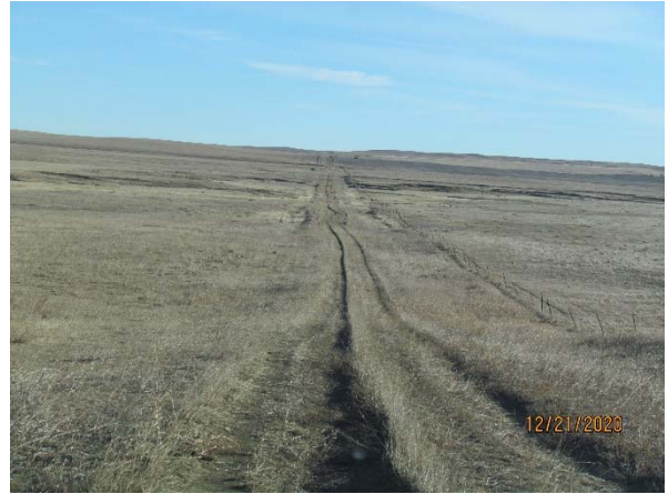
Photo 2: Section line (3 rd Avenue NE) roadway rutting, facing east.
