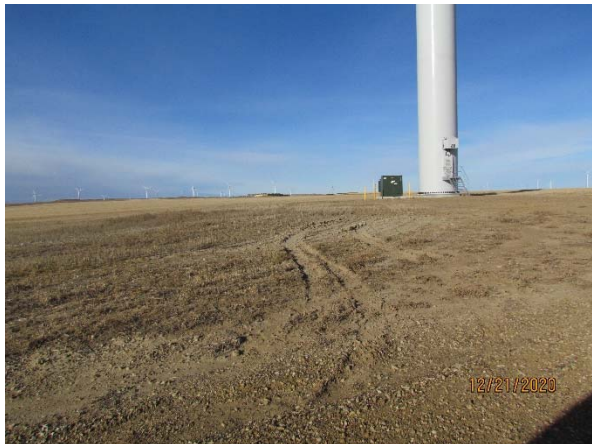
Photo 21: Tire rutting near Turbine 5.
