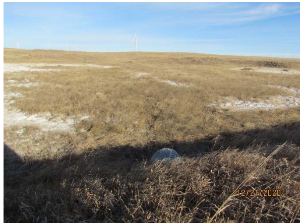
Photo 6: 3 rd Avenue NE stream crossing culverts, facing north.
