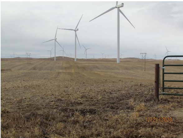
Photo 39: Turbines 14-16, no roadway access due to private property and gate.
