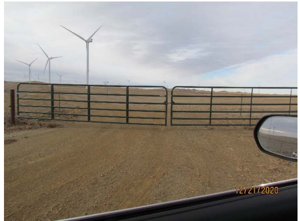
Photo 40: Turbines 14-16 private property and gate.
