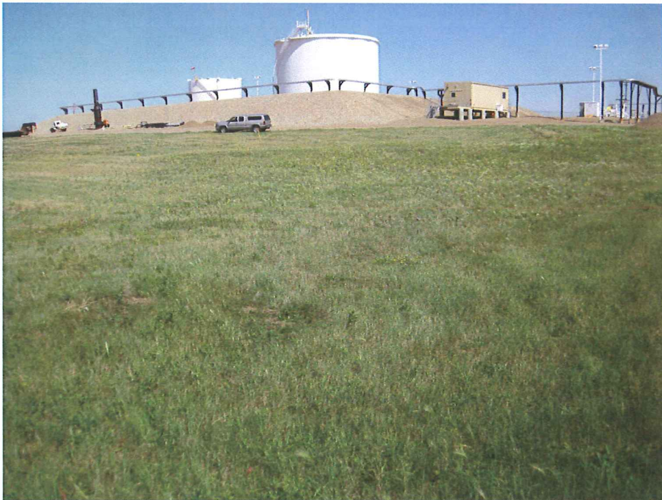
Figure 3: View inside the restricted area, looking northeast from the southwest corner (Image 7).
