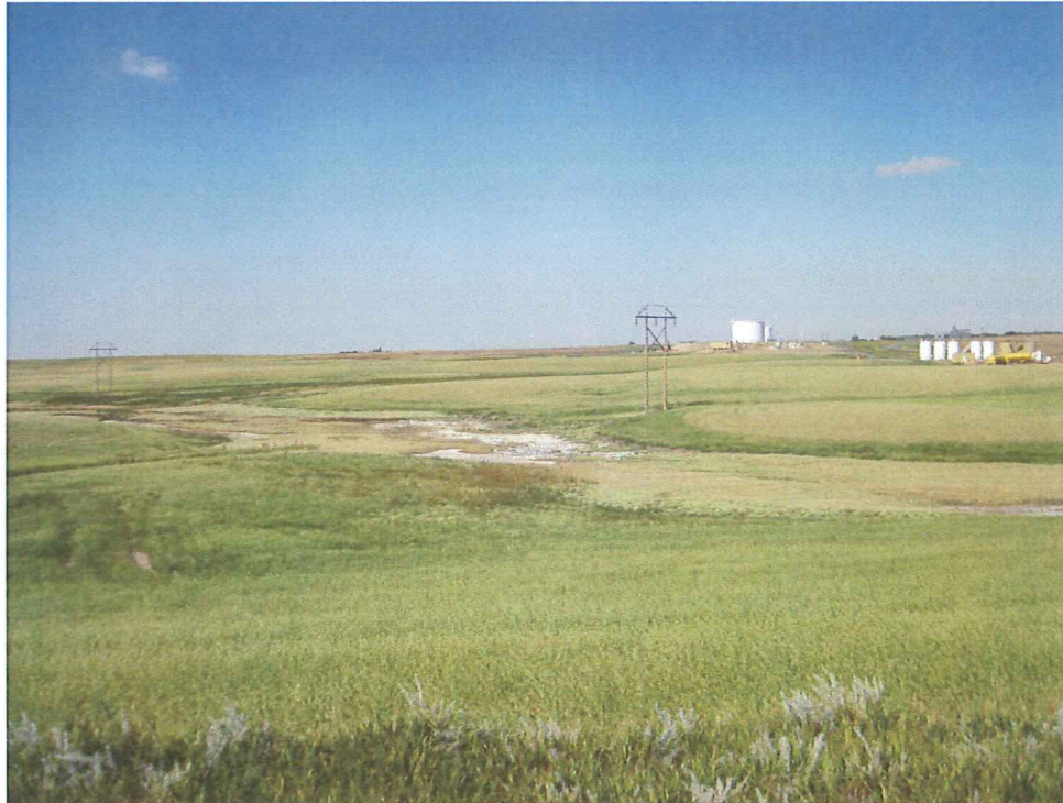
Figure 1: View over the APE looking north from the south side, the Grenora Station scheduled for expansion during the current project is visible in the background, and the older Grenora Station is visible on the east edge of the photo (Image 15).
