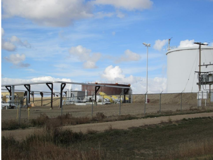
Photo 3. Direction: West. Storage tank and the associated structures after completion.
