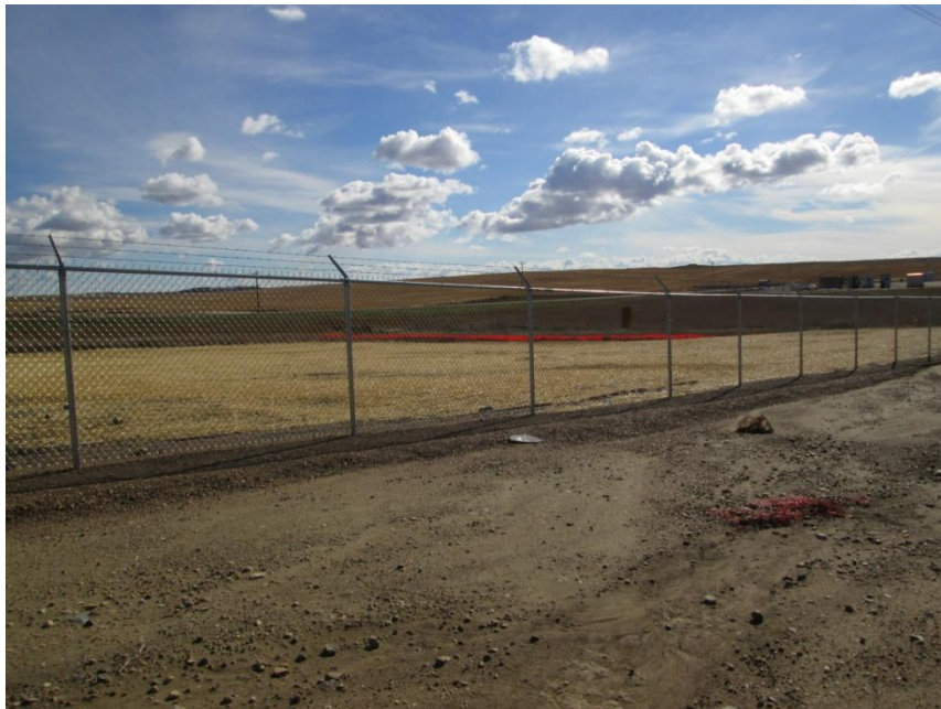
Photo 4. Direction: Southeast. Fiber blanket and silt fence in place prevent erosion and sedimentation of waterways.
