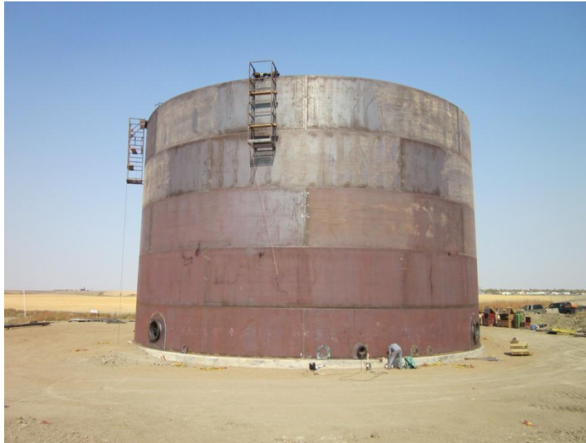
Photo 1. Direction: North. 40,000 Barrel Tank under construction during the September 2012 site visit.
