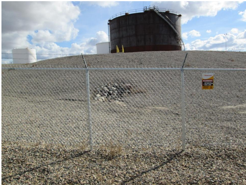
Photo 2. Direction: East. New Tank after completion during the October field survey. Note the culvert and rip-rap used for water and erosion control.
