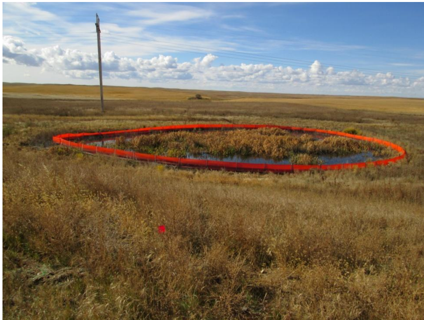
Photo 14. Direction: West. Natural wetland basins surrounded by a silt fence to prevent sediment migration.
