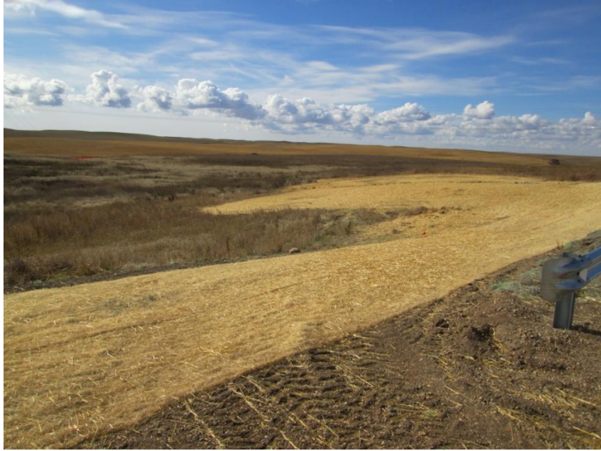
Photo 7. Direction: West/Southwest. Fiber blanket in place to prevent sedimentation of the wetland. The area has been reseeded and vegetation was just beginning to emerge from under the fiber blanket.
