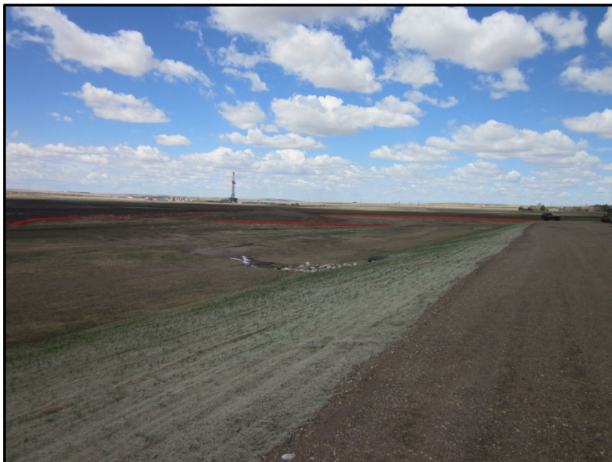
Photo 14. Direction: North. East edge of LACT lots showing erosion control measures in place and drainage set up along adjacent roadway.
