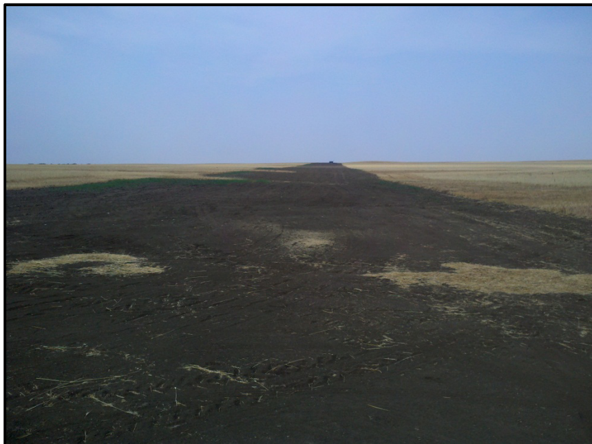
Photo 26. Direction: Northwest. Pipeline route northwest of East Fork Station.
