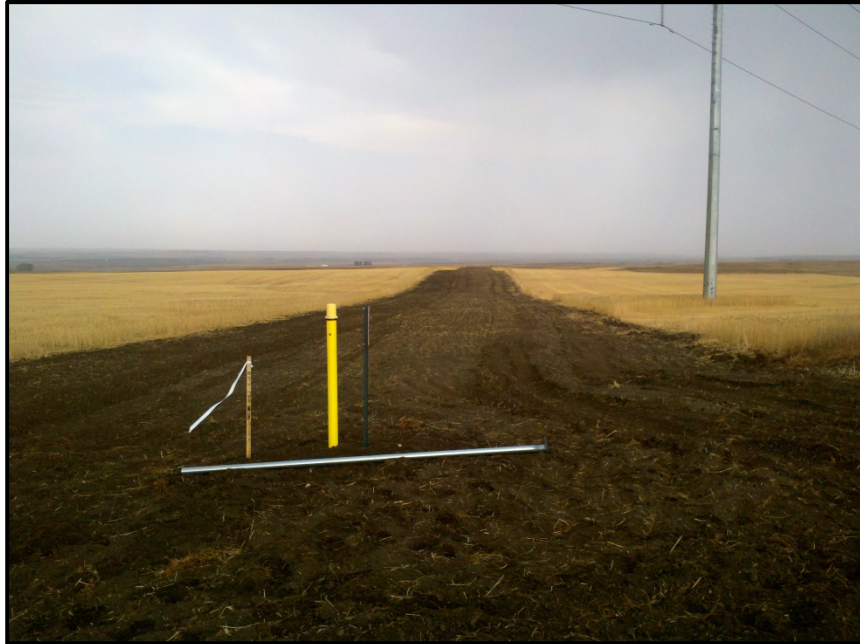
Photo 19. Direction: Northwest. Pipeline continued through cropland. Enbridge placed markers to show location of pipeline after backfilling, topsoil restoration, and general clean-up had been completed.
