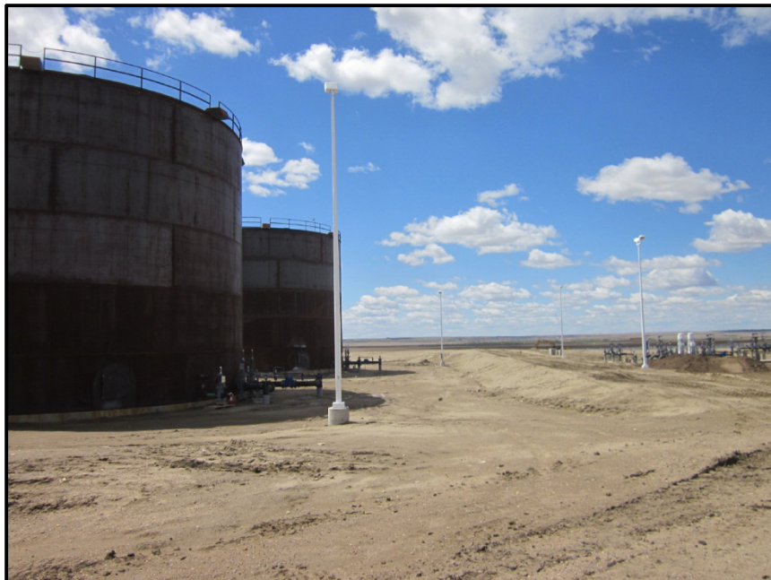
Photo 2. Direction: West. North end of tanks showing berm.
