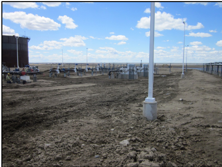
Photo 4. Direction: West. Another view of the tie-in area on north side.
