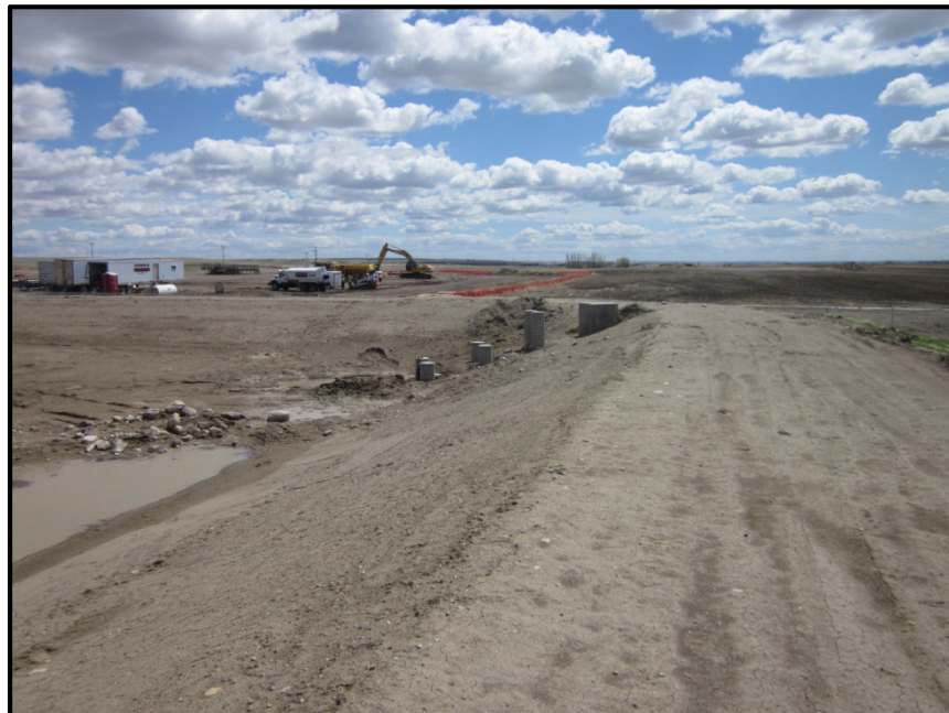
Photo 8. Direction: South. Drain valves within tank berm.
