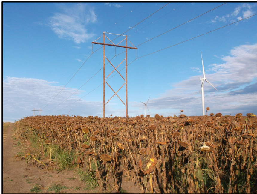
Photo 4. Direction: West. View of the transmission line as it spanned an agricultural area. No construction-related disturbance to the agricultural area was noted.
