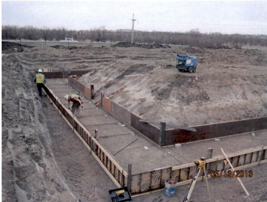
Forming Service Building Foundation (looking SW)
