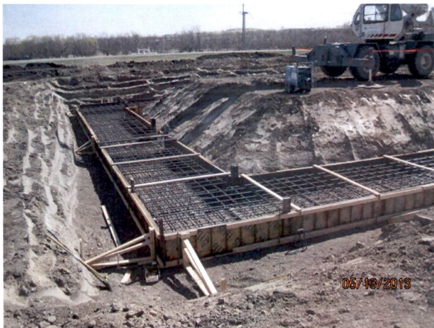
Rebar for Service Building Foundation (looking SW)
