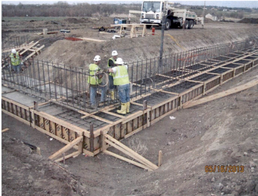
Placing concrete for Service Building Foundation (looking SW)
