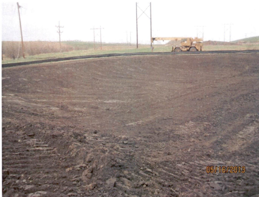
Stormwater Basin (looking NW)
