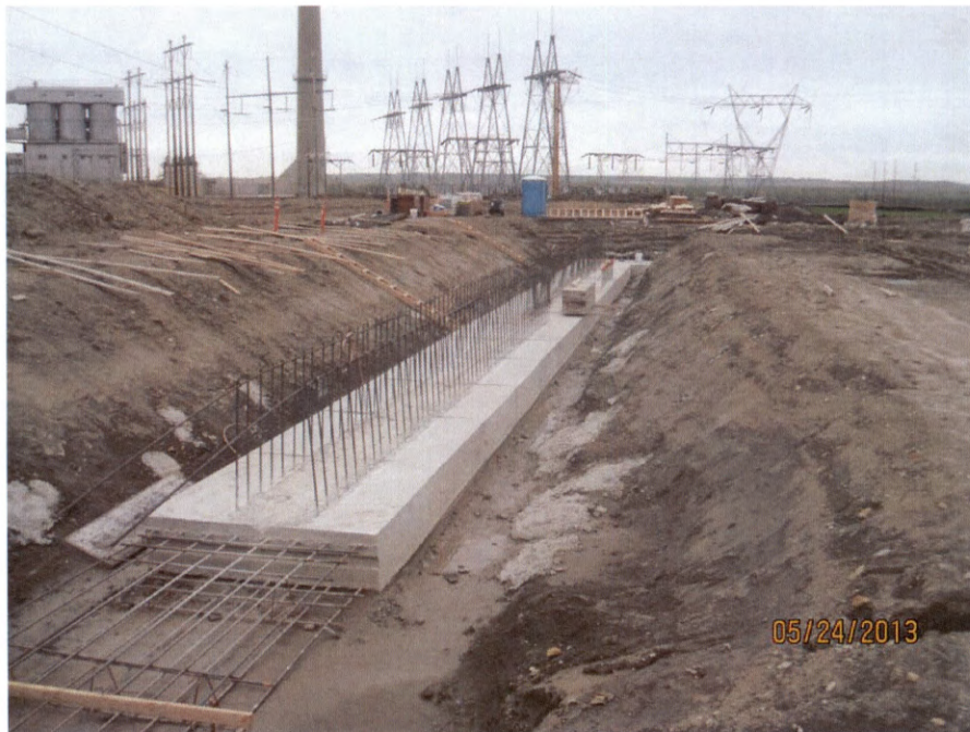
Service Building Foundation (NE)
