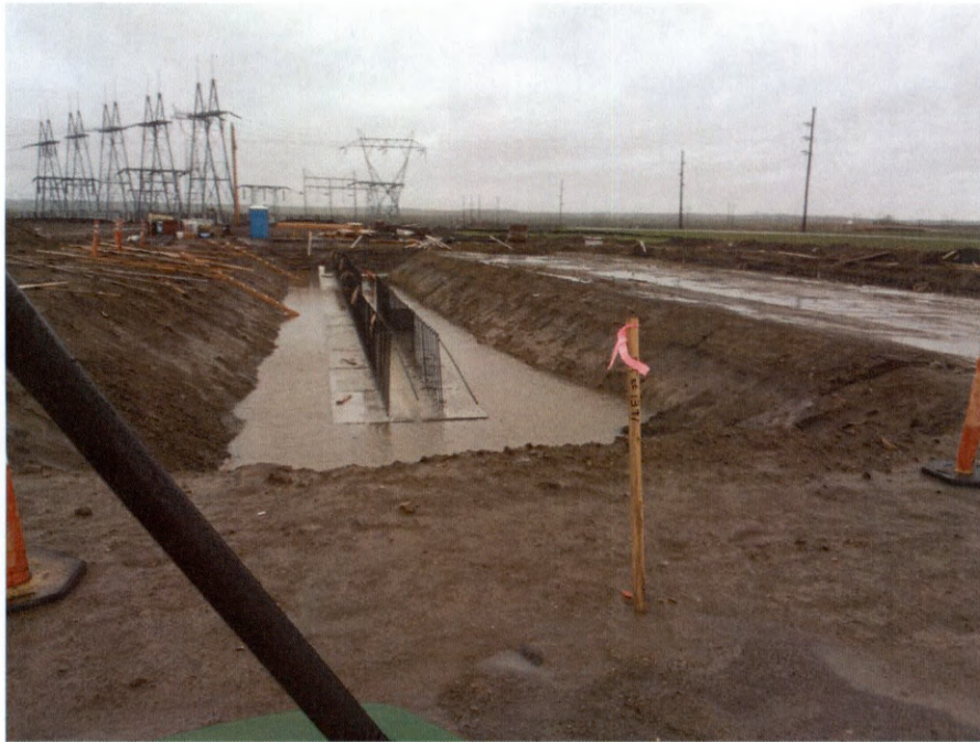
Service Building Foundation (E)
