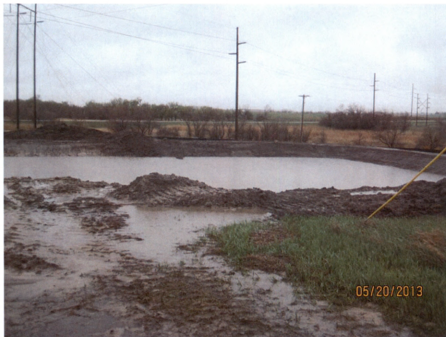
Stormwater Basin (looking S)
