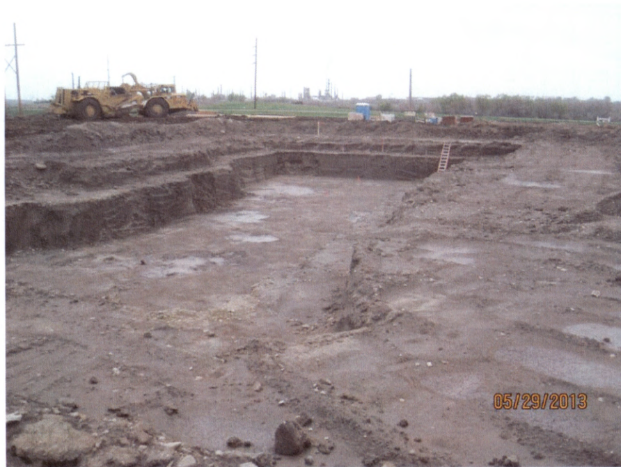
Turbine Foundation Excavation (looking SE)
