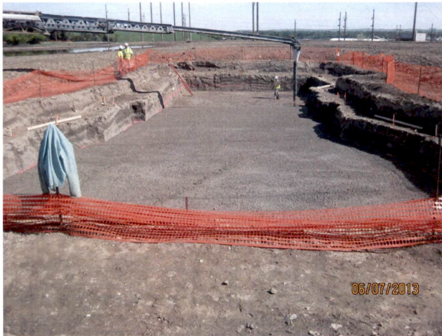
Turbine Foundation mud mat (looking N)
