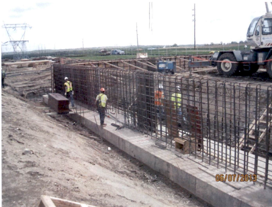
Service Building rebar (looking SE)
