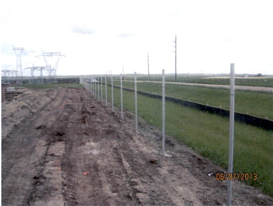
Site Security Fence Posts (looking E)
