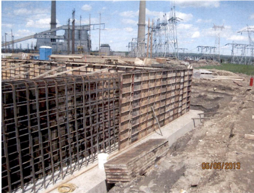
Service Building forms (looking NE)
